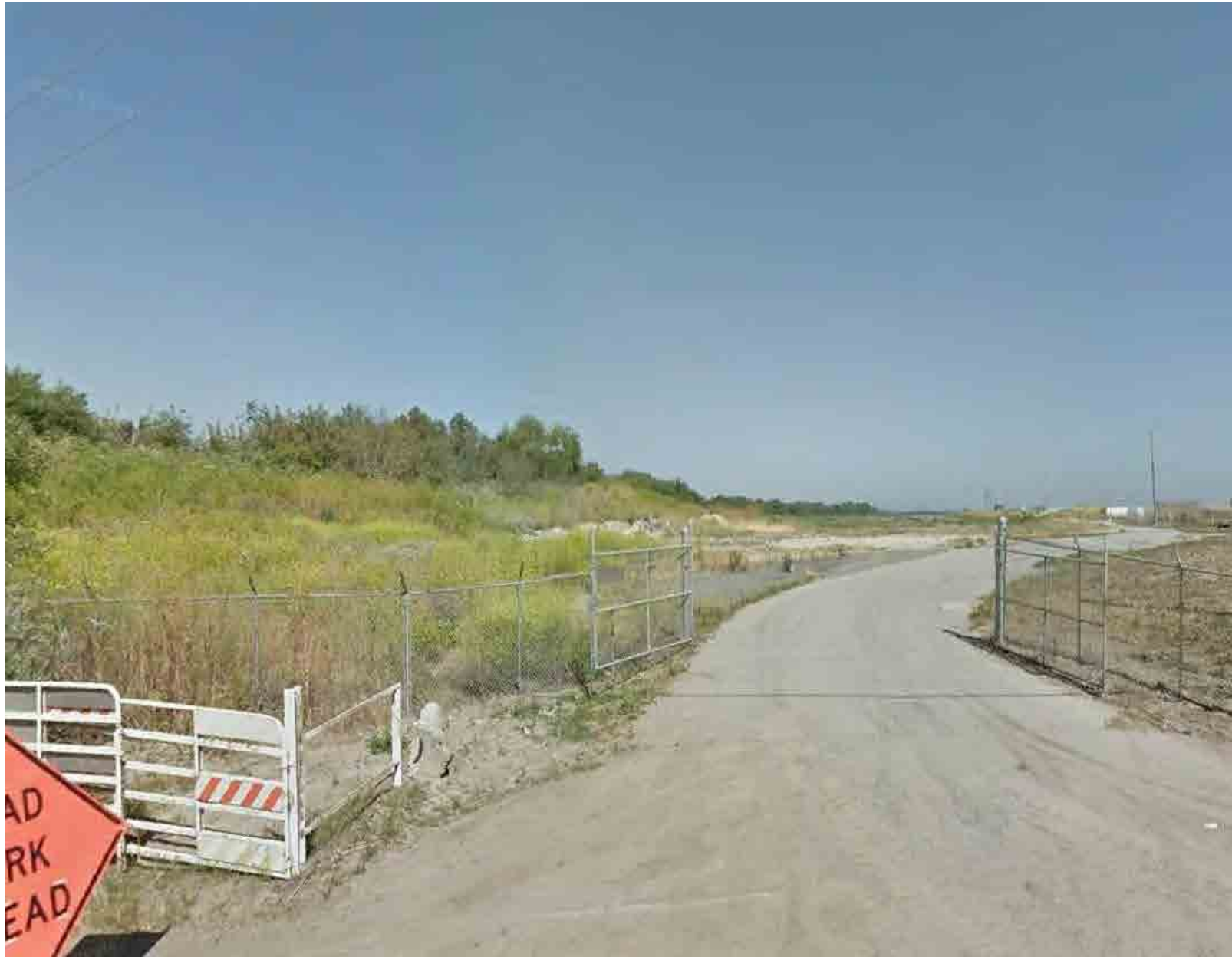
Figure 3. Salinas Treatment Facility entrance from Davis Road looking west
