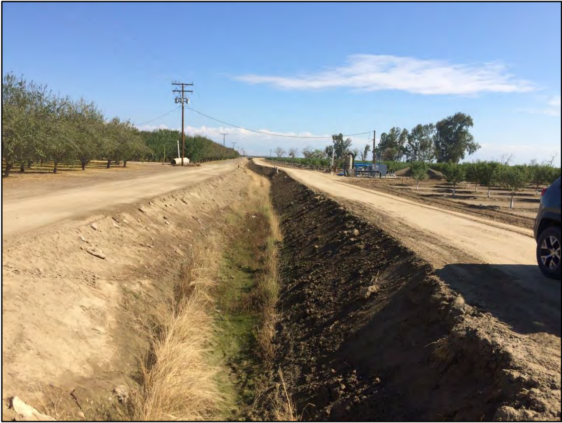
Photo Point 22: Facing east along ID1.
