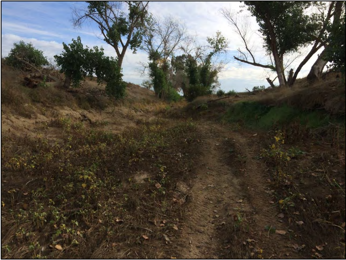
Photo Point 7: Facing to the east up the channel of Deer Creek.
