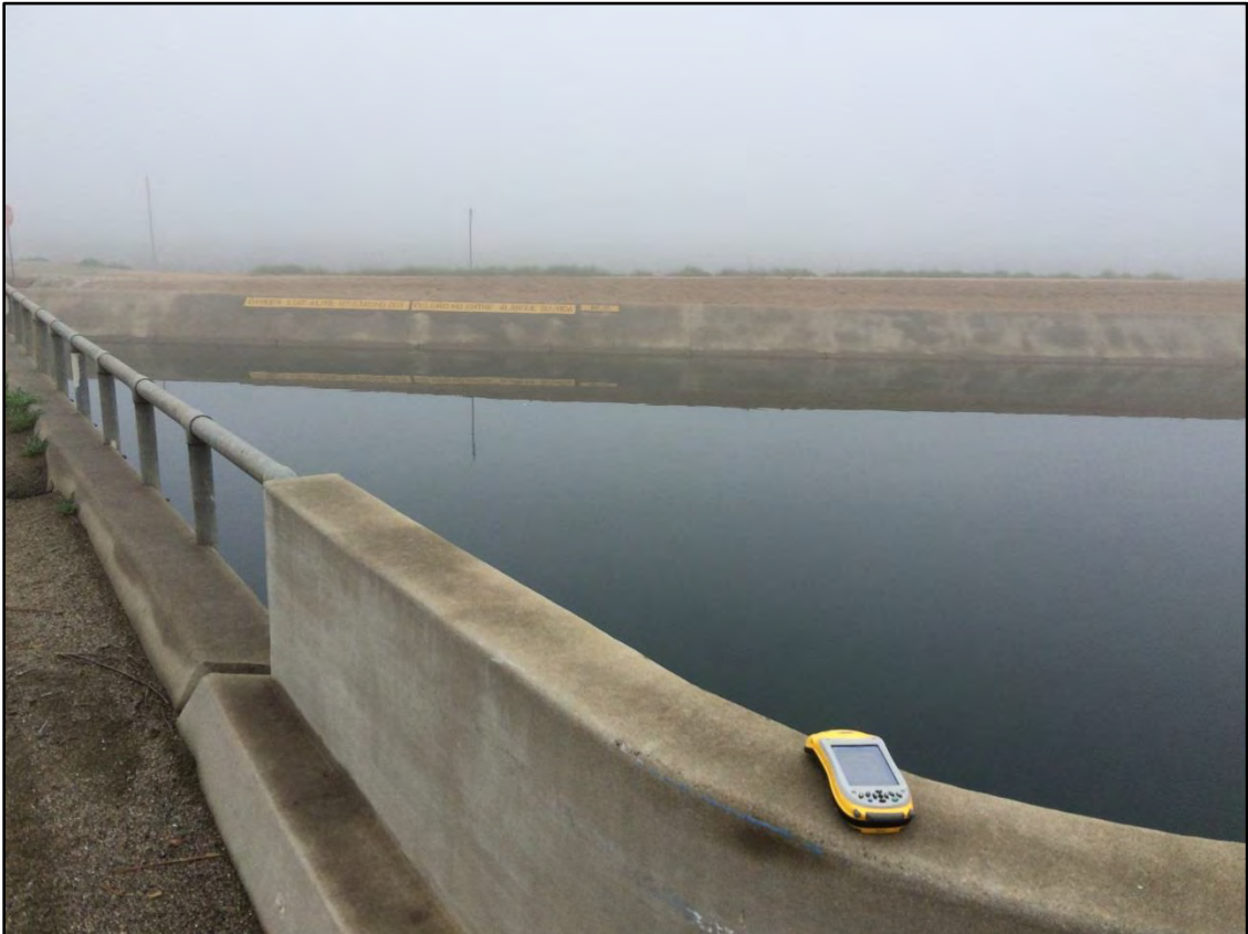
Photo Point 12 – Friant-Kern Canal Facing North
