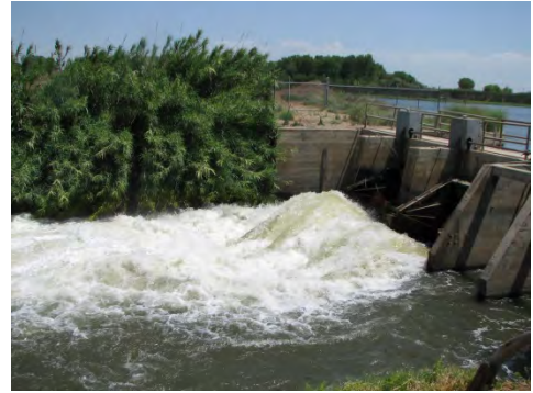
Headworks of the Main Canal
