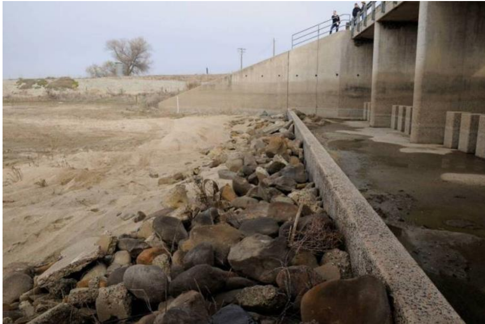
Figure 1-6. Concrete sill and bordering riprap along the downstream edge of the Chowchilla Bifurcation Structure in Reach 2B 3 (12/15/09)
