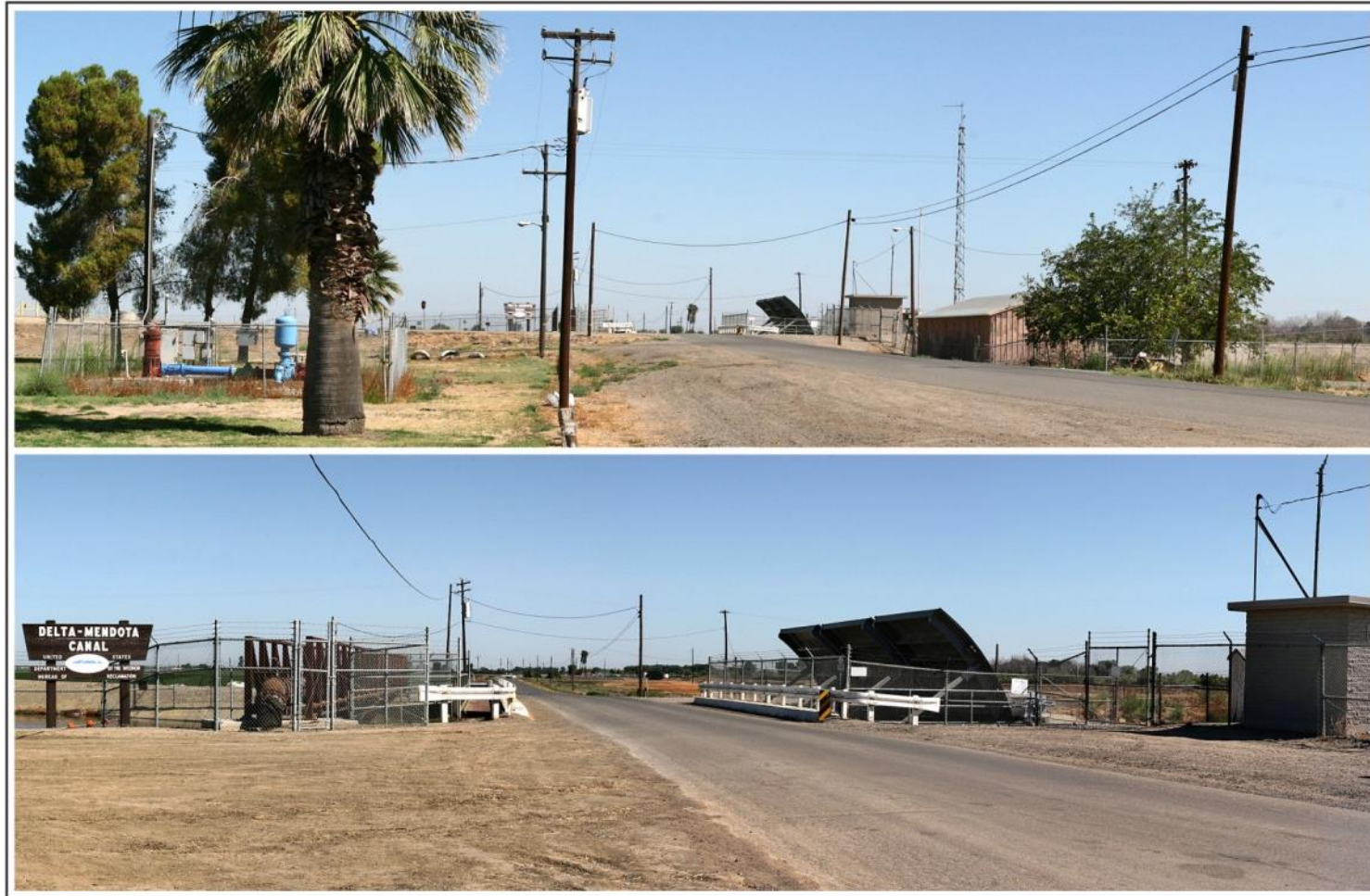
Figure 24-7. Two Views Looking North from Bass Ave. (Top): VP 8, within Mendota Pool Park and (Bottom): VP 9 at North Edge of Park along DMC
