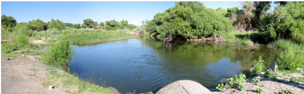
Note: Outlet of the ~5-foot diameter culvert is visible in the bottom-center of the photo and upstream edge of thick in-channel vegetation is visible in the background.
