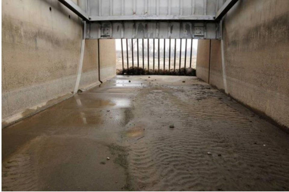
Figure 1-5. Inside of one of the bays at the Chowchilla Bifurcation Structure 2 (12/15/09)
