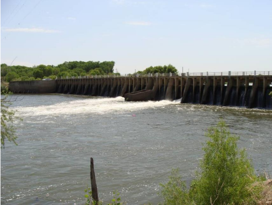
Figure 1-9. Downstream face of Mendota Dam (5/28/09)
