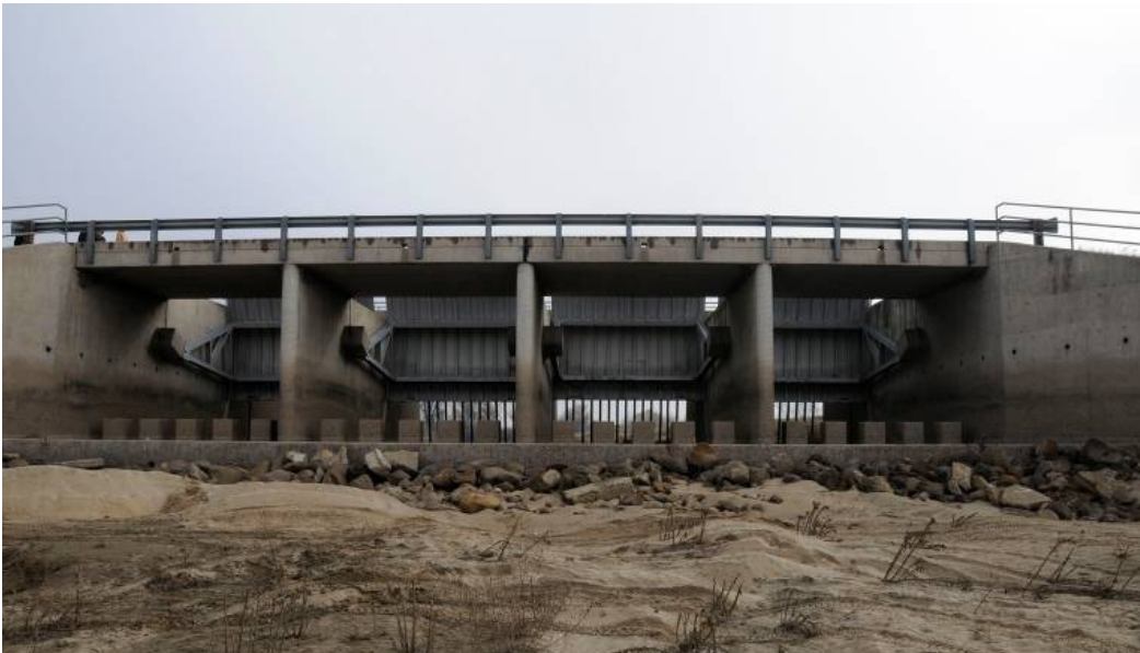
Figure 1-4. View from downstream of the Chowchilla Bifurcation Structure in Reach 2B (12/15/09)
