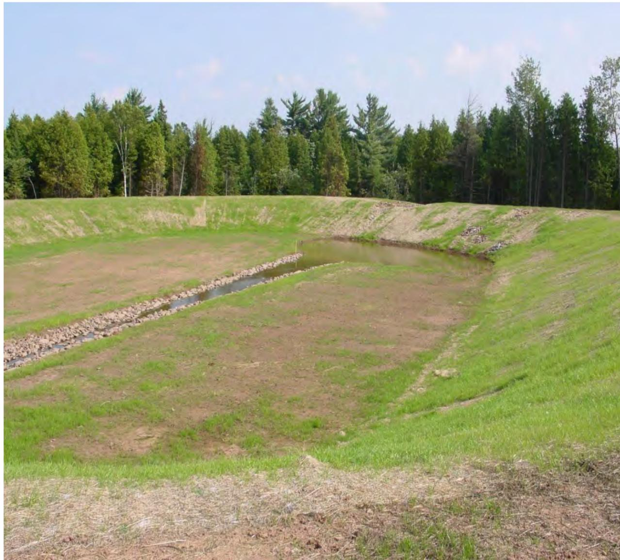
A *detention pond* (left) is a low lying area that is designed to temporarily hold a set amount of water while slowly draining to another location.
