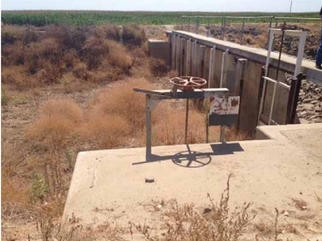
Photograph #7 (above). Another turnout is proposed adjacent to this existing turnout on Deer Creek.
