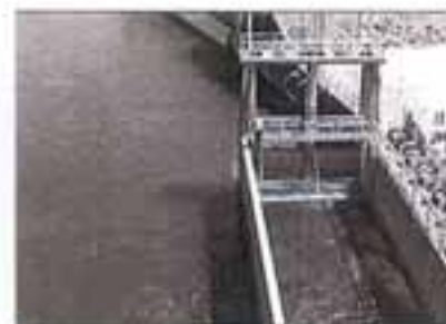
View of surface flow conditions exiting the right bank fishway.
