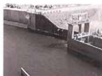
View of surface flow conditions downstream of the right bank fishway.
