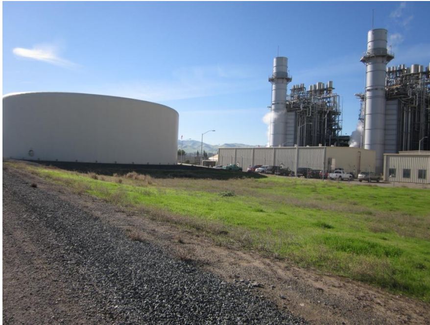
View looking south at an existing storage tank. The DEC is to the right (west)
