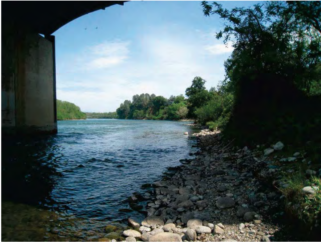
Figure A-8. Looking downstream (river right) under the Market Street bridge.
