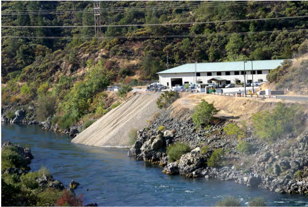
Figure A-3. Keswick gravel augmentation site following 15,000 tons placed in 2012, looking downstream.
