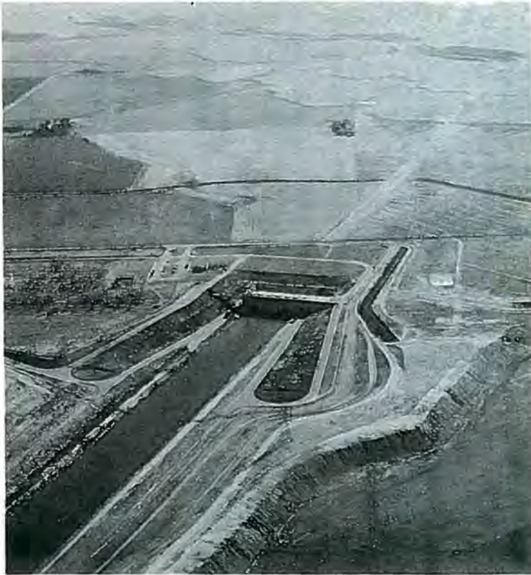
Tracy Pumping Plant
