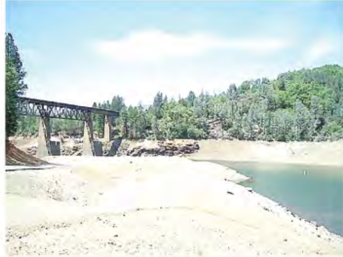
Sacramento Arm VAU, KOP 14, Photo 14b View looking northwest from Lower Salt Creek Road at the Salt Creek Resort.
