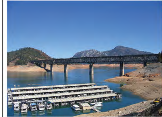
Bridge Bay VAU, KOP 2, Photo 2 View of the I-5/Pit River Bridge from Bridge Bay.
