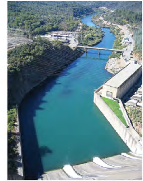
Shasta Dam VAU, KOP 2, Photo 2b View of the Shasta Dam spillway and the upper Sacramento River from Shasta Dam.
