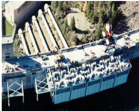
Figure 2-4. TCD Located on Upstream Face of Shasta Dam
