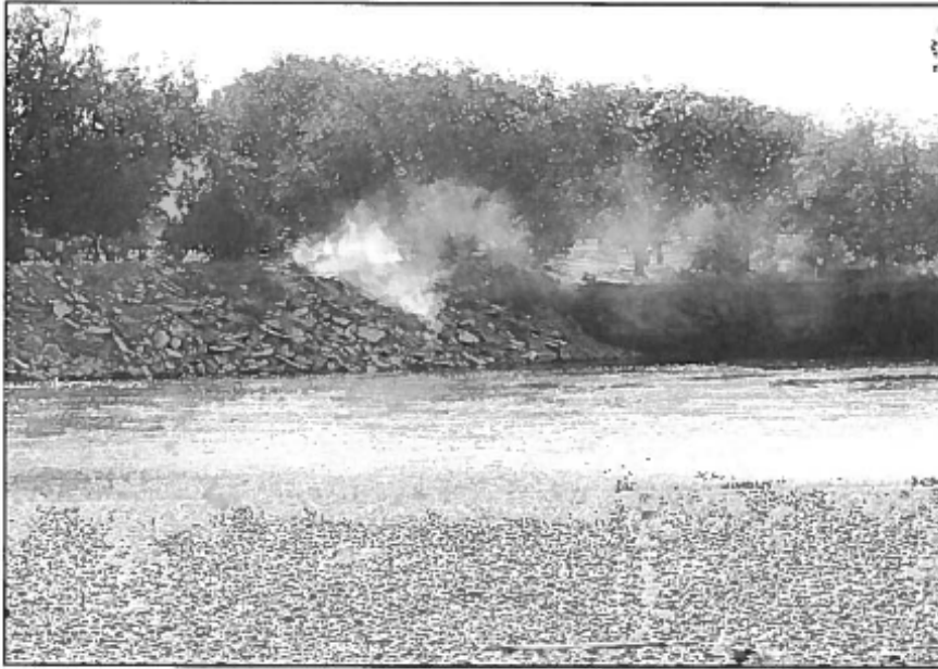
Figure 12. Private revetment being placed on an eroding bank on the middle Sacramento River. Photo by Dave Forwalter (DWR, Northern Region Office), 2007.
