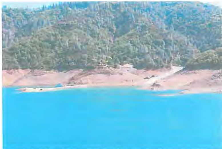
Figure 9: "Bathtub Ring" from Shasta Dam, 9-20-2013
