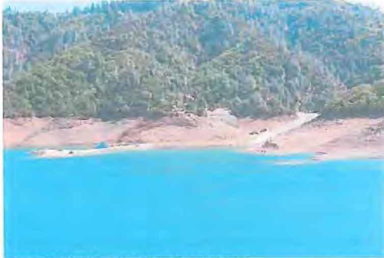
Figure 9: "Bathtub Ring" from Shasta Dam, 9-20-2013
