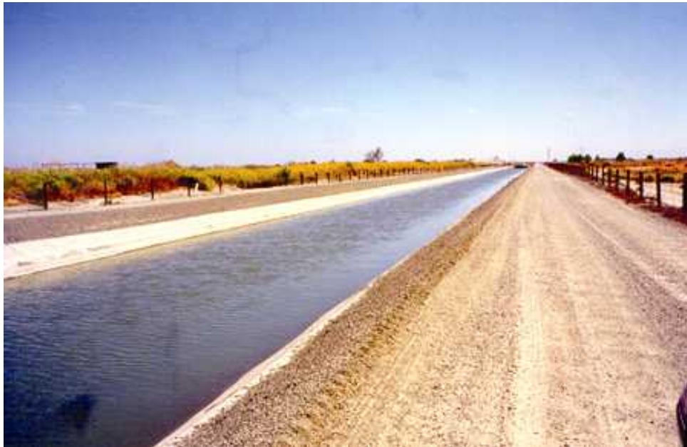
Figure 16-3 Existing San Luis Drain
