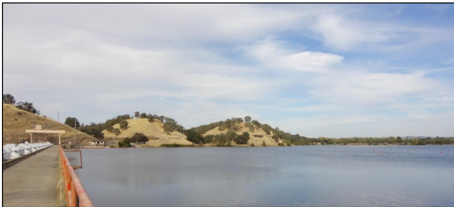
Photo 2: View north of the northern bank of the American River from Nimbus Dam.
