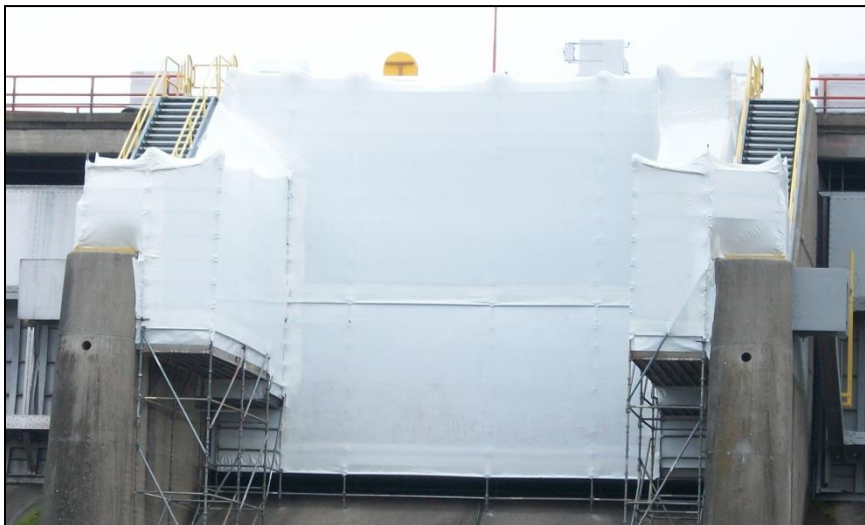
Photo 2: Poly Sheeting Containment
