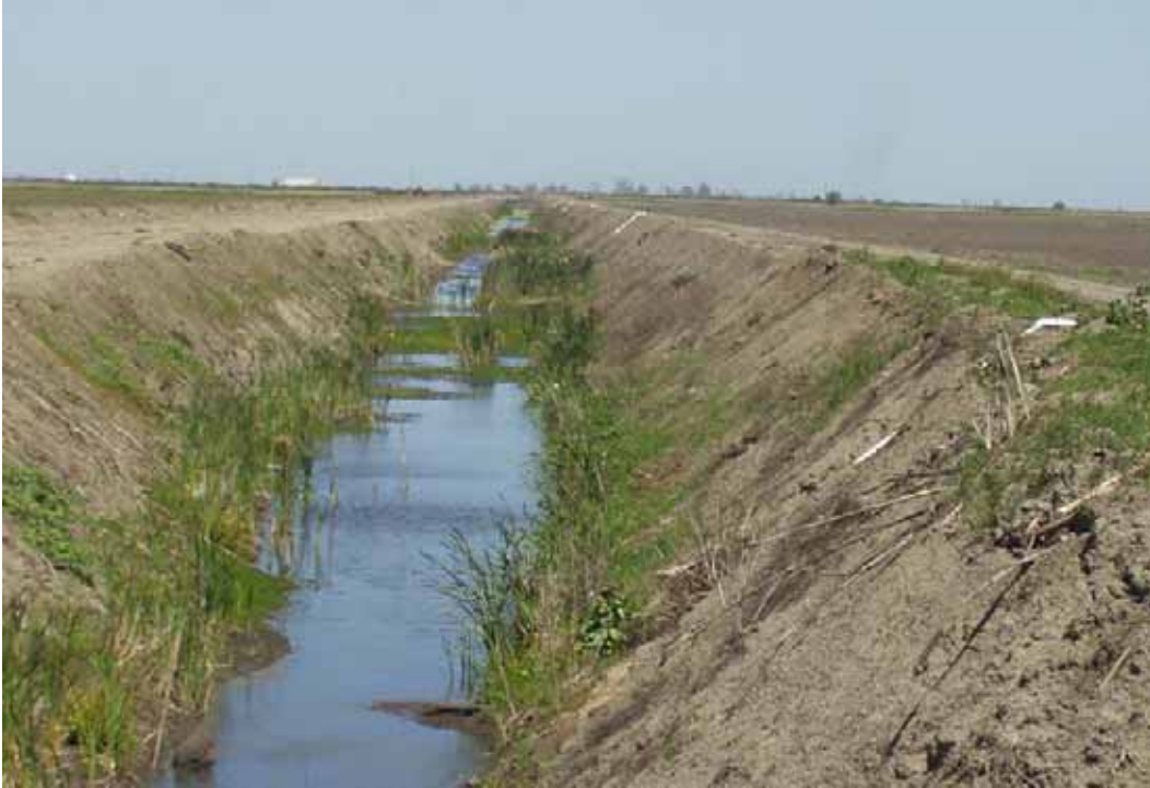
Typical drainage ditch on Victoria Island with scant freshwater marsh, aquatic vegetation, and open water (April 18, 2005)
