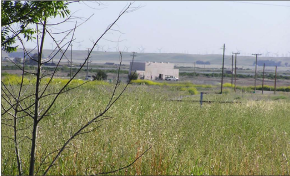
View of Mallard Slough Intake and Pump Station, facing northeast (April 18, 2005)
