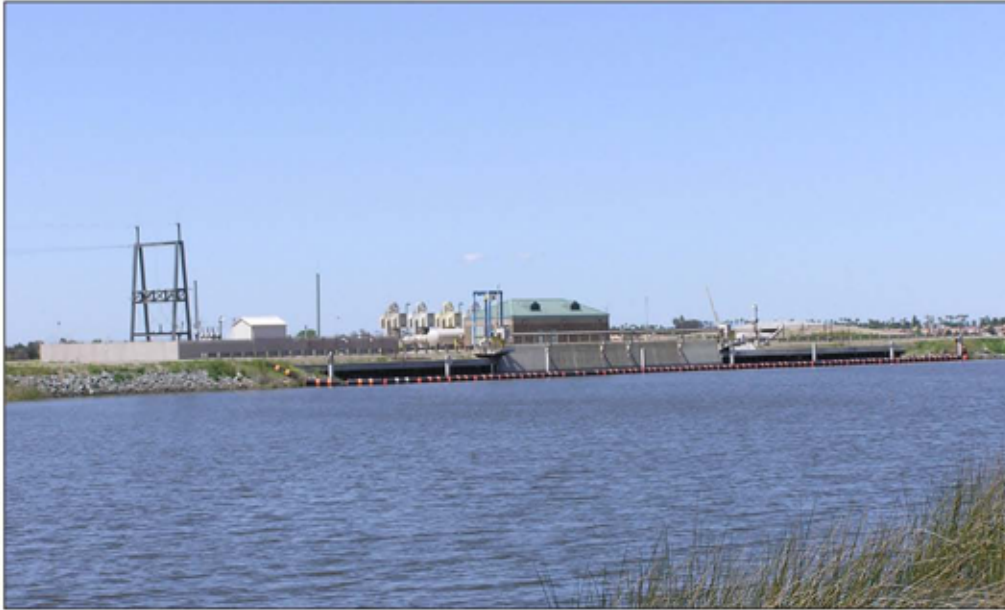
View of Old River Intake and Pump Station from the levee road on Victoria Island, facing northwest (April 18, 2005)
