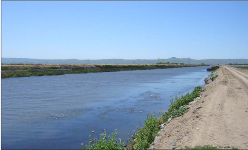
View of Victoria Canal (potential intake locations) from the levee road on Victoria Island, facing southwest (April 18, 2005)
