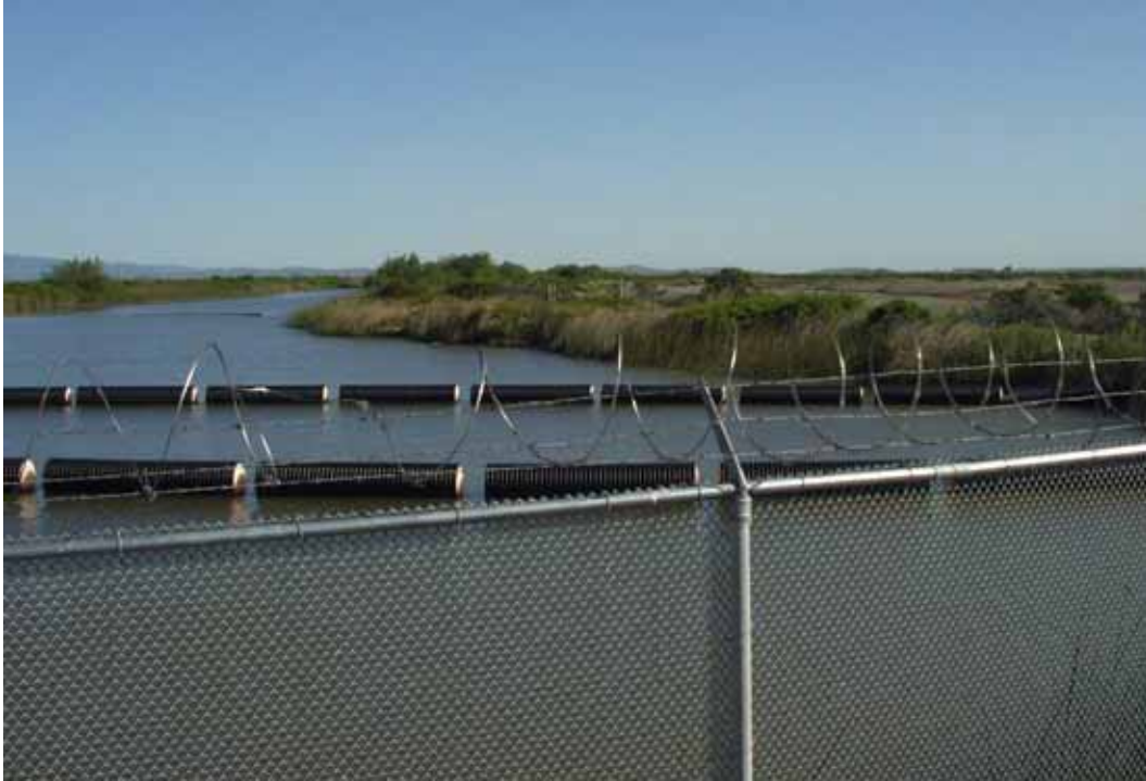
Coastal brackish marsh and riparian scrub communities at existing Mallard Slough Intake and Pump Station (April 18, 2005)
