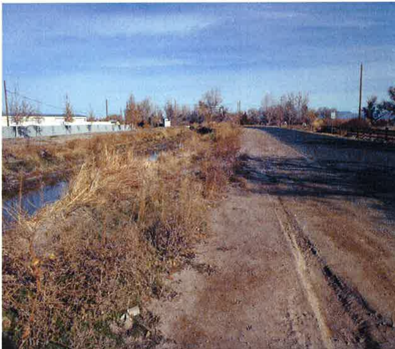
Photograph 1. Acquired Portion Owned in Fee Title SWG Pipeline Abandonment and Replacement at V Line Canal
