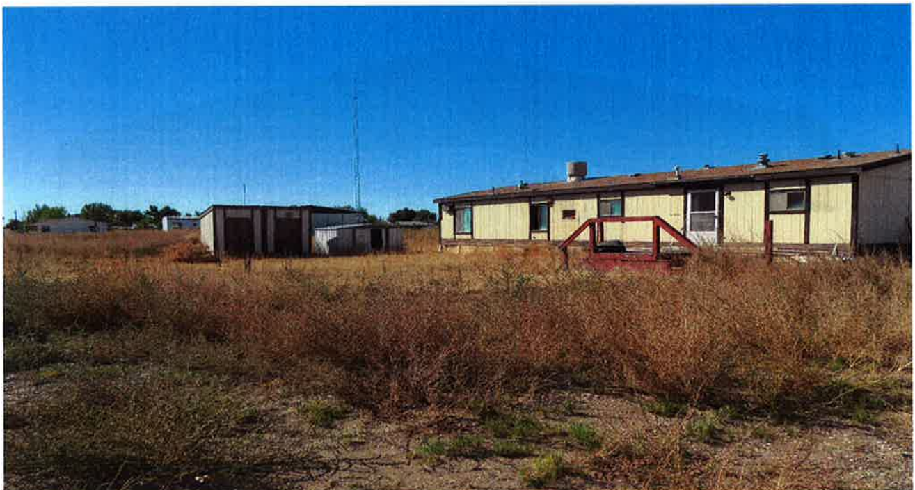
Figure 4 - Looking at Modular Building to the Right with two Storage Sheds on Left
