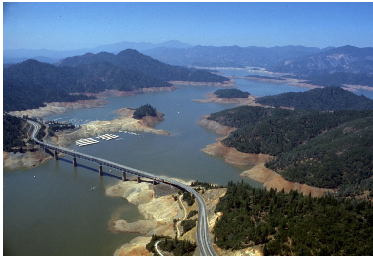
Figure 3.14-10. The "Bathtub Ring" Effect at Shasta Reservoir
