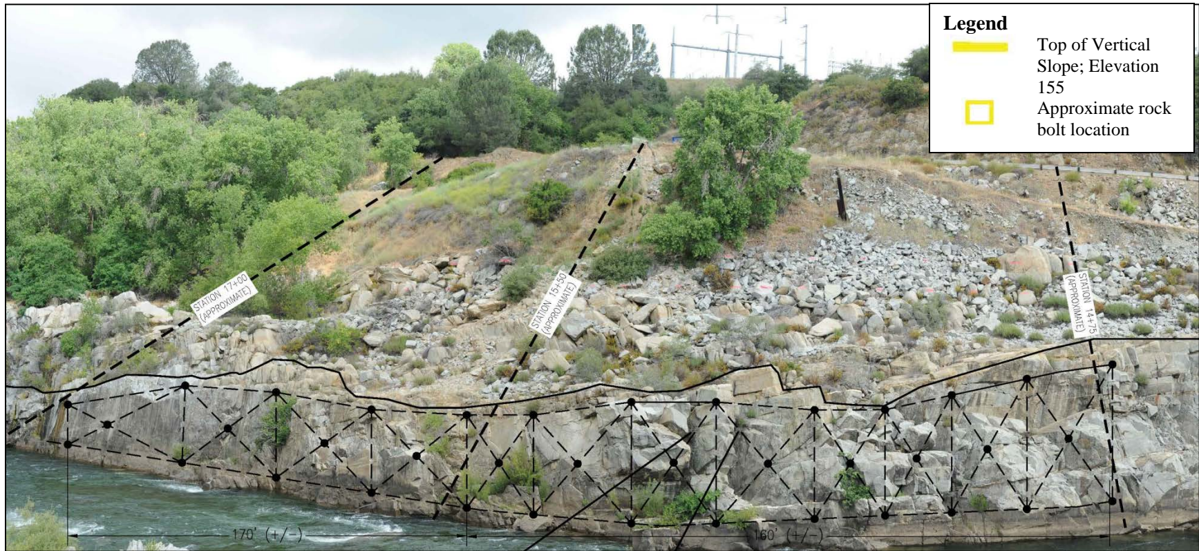
Figure 3. Approximate Rock Bolt Locations
