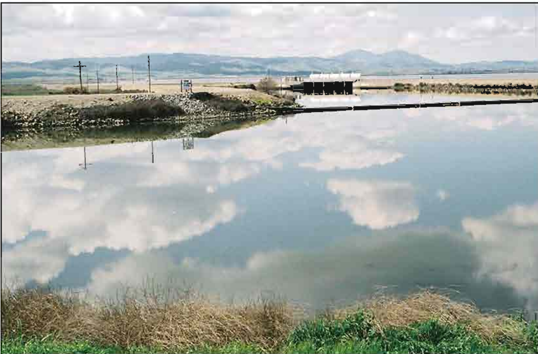
Photograph 7.6-12. West Canal Dredging Site View is west to Coastal Range.
