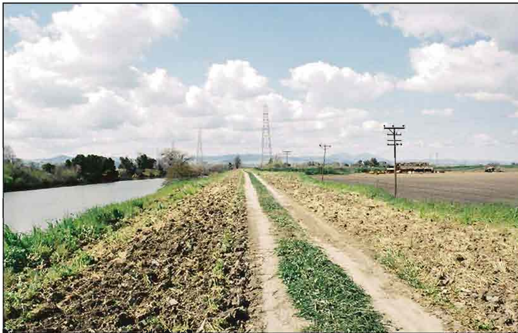
Photograph 7.6-8. Grant Line Canal Gate Site View is west from the northern levee.
