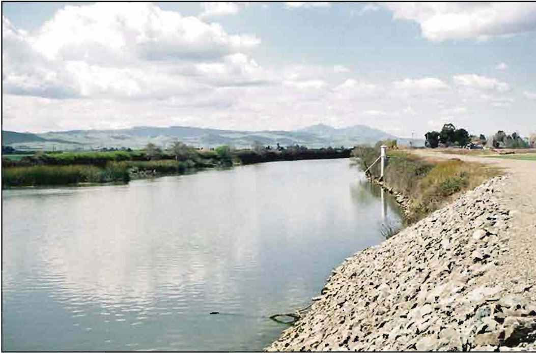
Photograph 7.6-11. Old River Gate Site View is southwest from the northern levee.
