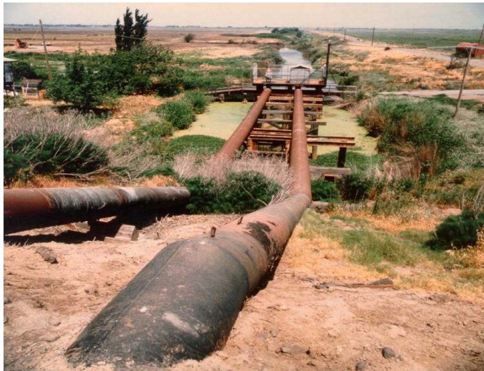
Photograph 5.3-10. Drainage Pumps on Twitchell Island That Returns Stormwater Runoff and Agricultural Drainage Flows to the Delta Channels (Source: California Department of Water Resources.)
