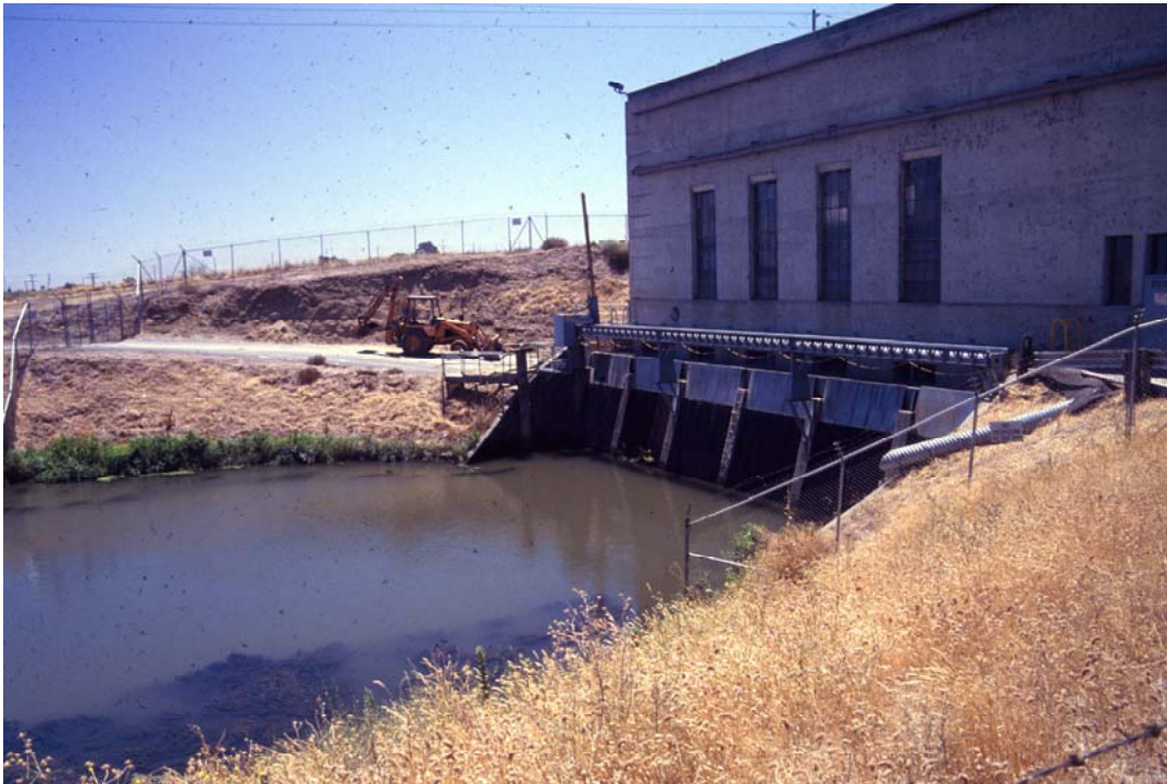
Photograph 5.3-7. Contra Costa Water District Pumping Plant #1 Near Oakley Capacity of 350 cubic feet per second, completed in 1940 with deliveries to Pittsburg. (Source: Bureau of Reclamation.)
