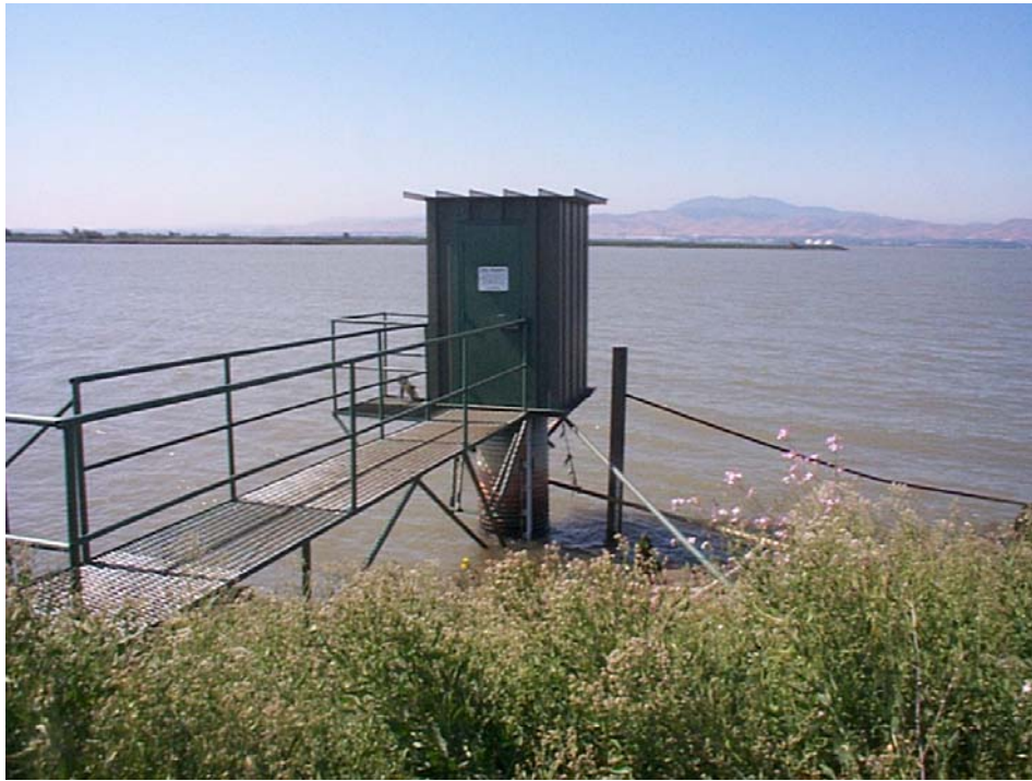
Photograph 5.3-1. Collinsville Salinity (EC) Monitoring Station Looking south across the Sacramento River toward the confluence of the San Joaquin River, with Mt. Diablo in background. (Source: California Department of Water Resources.)
