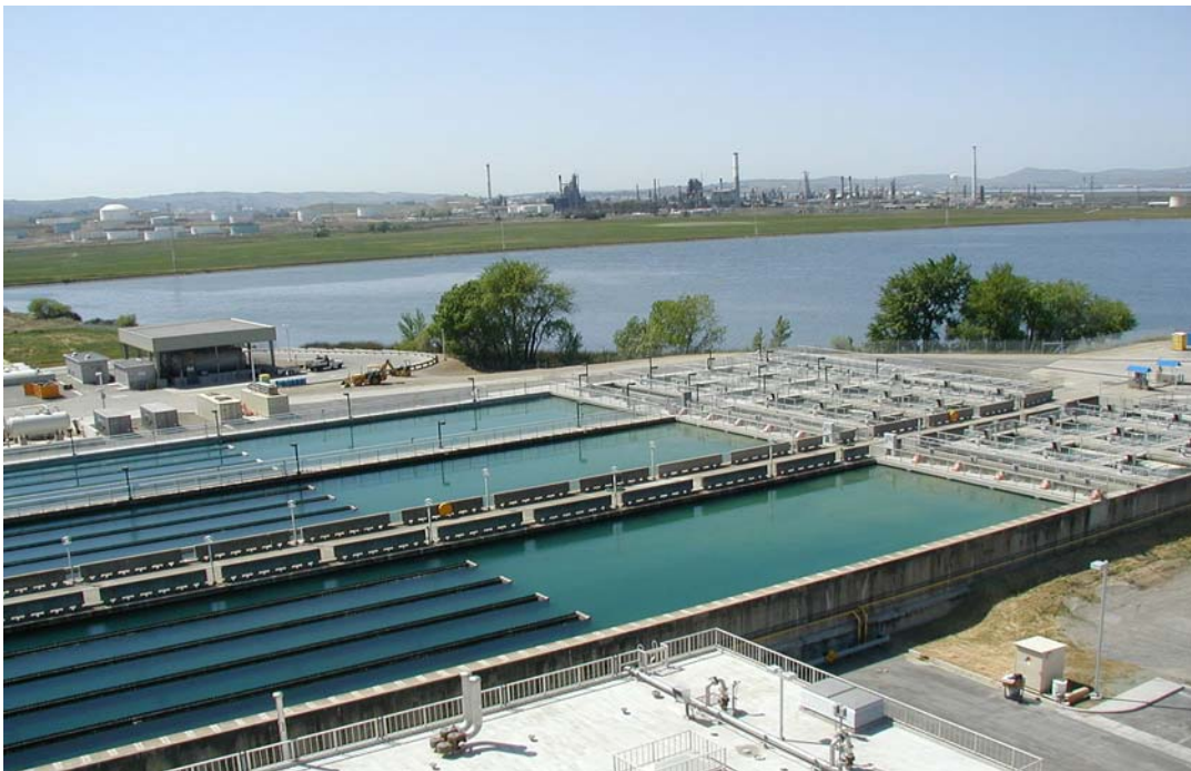
Photograph 5.3-8. Contra Costa Water District Bollman Water Treatment Plant Sedimentation Basins and Mallard Reservoir Contra Costa Canal supplies the raw water to Mallard Reservoir, where it is stored until treatment. (Source: Contra Costa Water District.)
