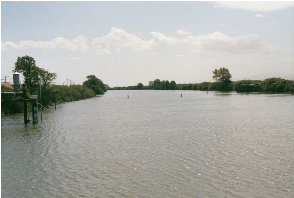
Photograph 5.2-46. Grant Line Canal Looking East (Upstream) from Temporary Barrier Site with Two Agricultural Diversion Pumps (March 4, 2003)
