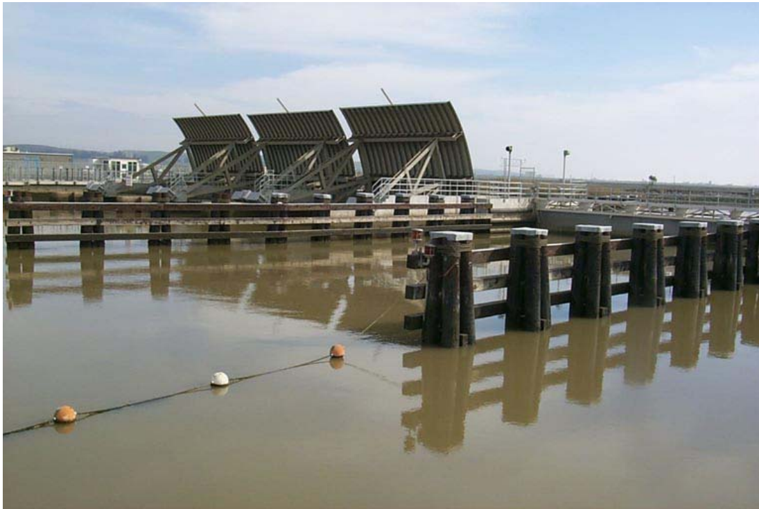
Photograph 5.2-47. Suisun Marsh (Montezuma Slough) Salinity Control Gates in Open Raised Position (Source: California Department of Water Resources Interagency Ecological Program.)
