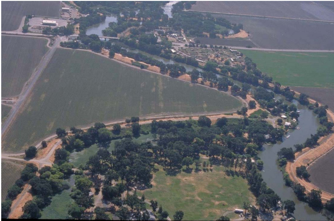
Photograph 5.2-37. Tracy Boulevard Bridge Crossing the Old River Channel, Looking East The Tracy Wildlife Club is at the bottom of the photo. (Source: California Department of Water Resources.)
