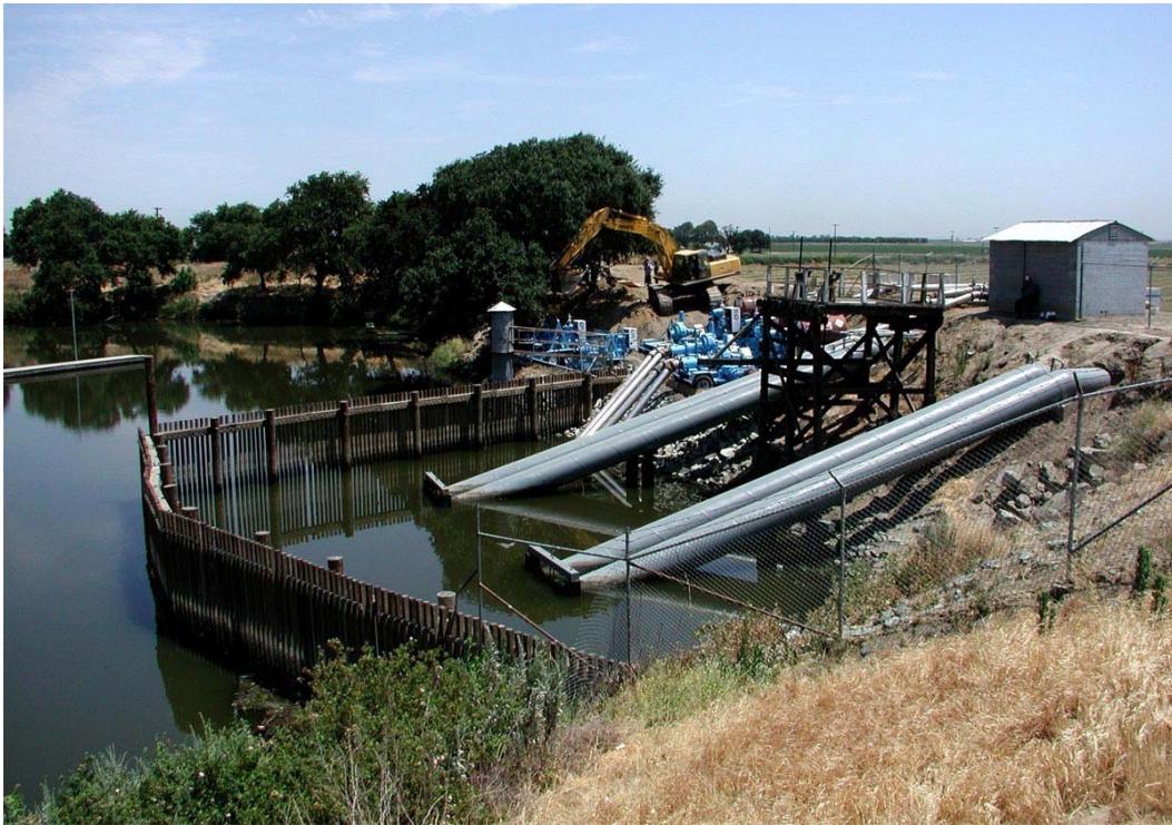
Photograph 5.2-29. Siphons That Supply Tom Paine Slough, Located in Sugar Cut off Old River East of Tracy Boulevard Bridge Temporary pumps were installed in summer 2003. (Source: California Department of Water Resources.)
