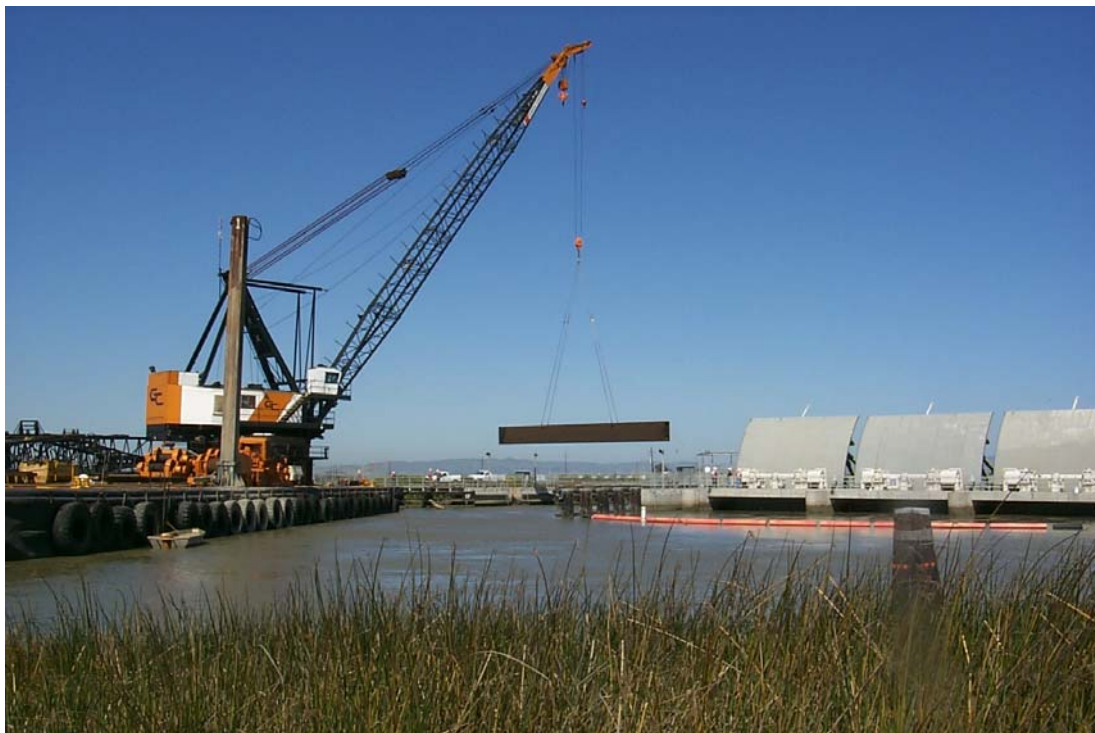
Photograph 5.2-48. Suisun Marsh (Montezuma Slough) Salinity Control Gates Flashboard Removal (Source: California Department of Water Resources Interagency Ecological Program.)
