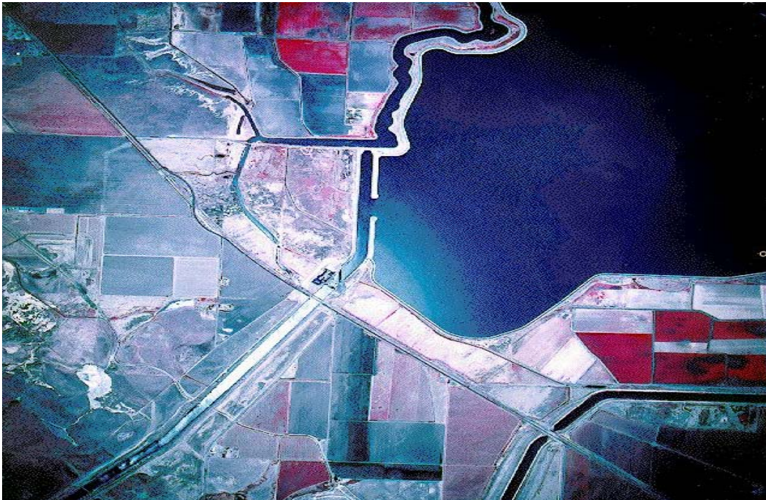
Photograph 5.2-31. West Side of Clifton Court Forebay with John E. Skinner Fish Salvage Facility (Center)
