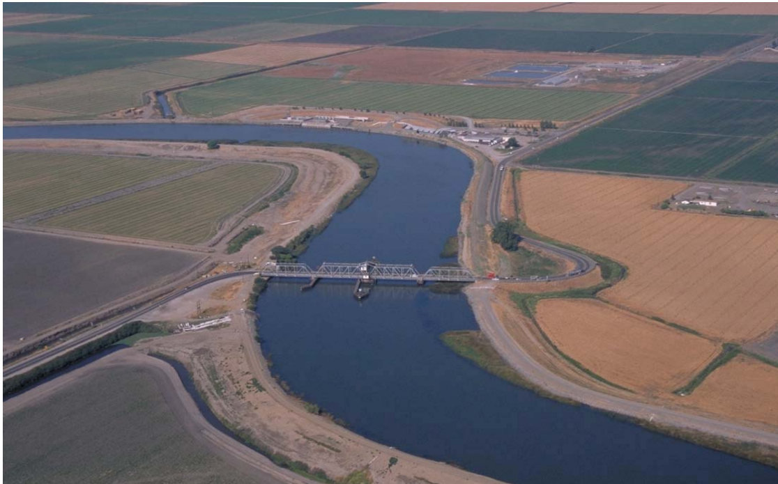
Photograph 5.2-36. State Route 4 Bridge over Old River Just North of Los Vaqueros Pumping Plant (Source: California Department of Water Resources.)
