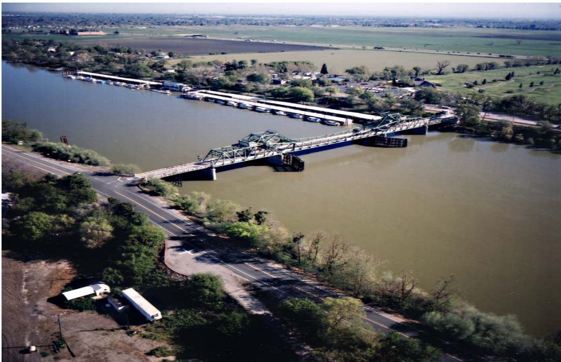
Photograph 5.2-6. Sacramento River at Freeport Bridge, South of Sacramento A USGS tidal flow meter was installed here in 1980 to measure tidal flow to regulate Sacramento Regional Wastewater treatment plant effluent discharge mixing. (Source: California Department of Water Resources.)
