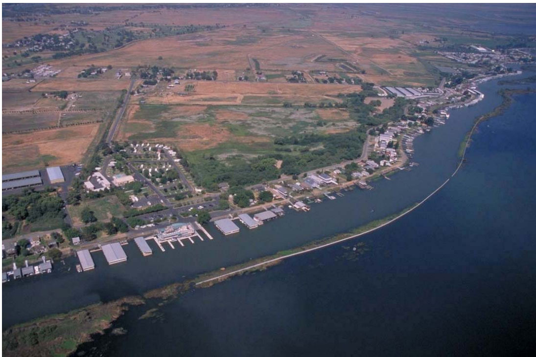
Photograph 5.2-14. Seawall along the Southwest Franks Tract Levee along Bethel Island (Source: California Department of Water Resources.)
