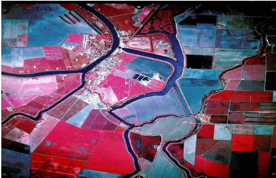
Photograph 5.2-7. Aerial View of Sacramento River Bend, Looping in Upper Left of Photo, at Walnut Grove
