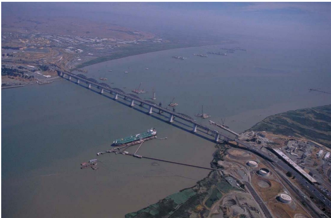
Photograph 5.2-2. Interstate 680 Martinez Bridge Looking East toward Suisun Bay (Source: California Department of Water Resources.)
