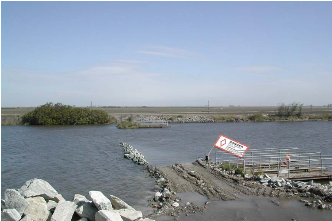
Photograph 5.2-41. Middle River Temporary Barrier Site Looking South across Union Island The center section has not been installed yet. Culvert sections on both banks are not removed during the winter. (Source: California Department of Water Resources.)
