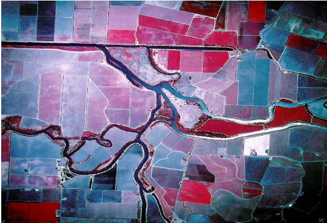
Photograph 5.2-23. Aerial View of East End of Grant Line Canal (Top), Old River from Head of Old River (East) toward Tracy Boulevard Bridge to West (Just off Photo), with Tom Paine Slough Siphon Station off Sugar Cut (Bottom) (Source: University of California, Berkeley.)
