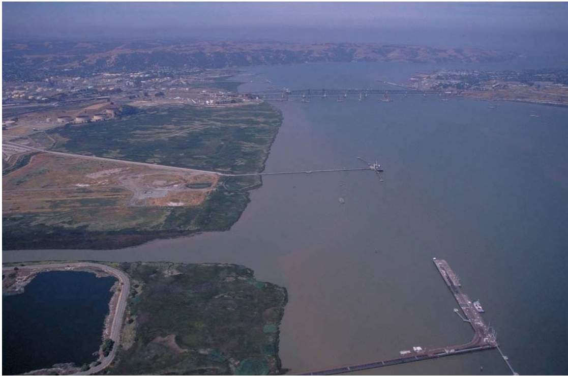
Photograph 5.2-1. Looking West toward Carquinez Strait with Benicia to South (Left) and Martinez to North (Right) (Source: California Department of Water Resources.)
