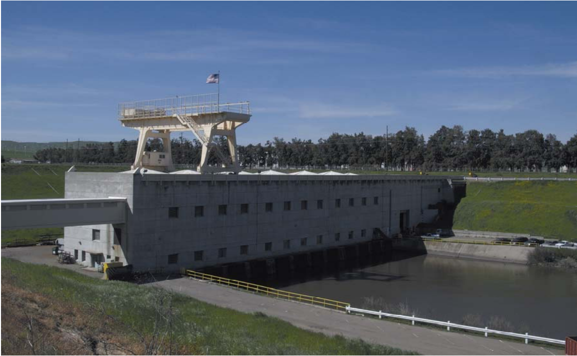
Photograph 5.1-15. CVP Tracy Pumping Plant (Source: Bureau of Reclamation.)
