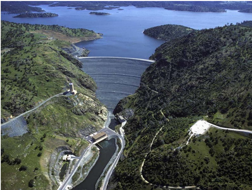
Photograph 5.1-I4. New Melones Dam (Source: Bureau of Reclamation.)
