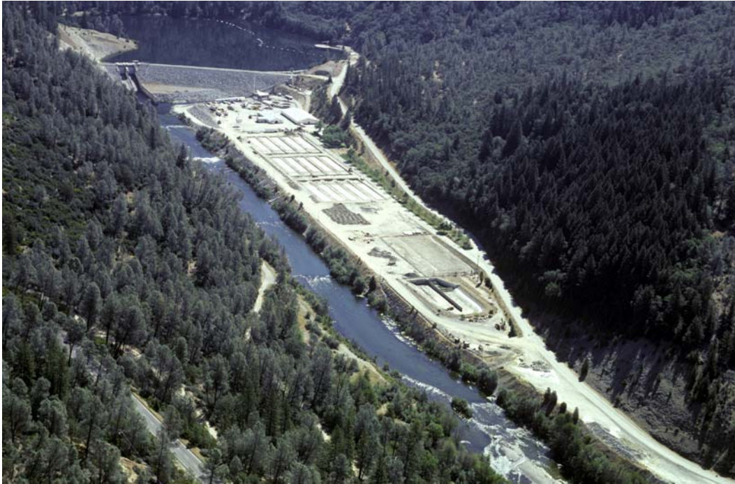
Photograph 5.1-2. Lewiston Dam and Lewiston Hatchery (Source: Bureau of Reclamation.)
