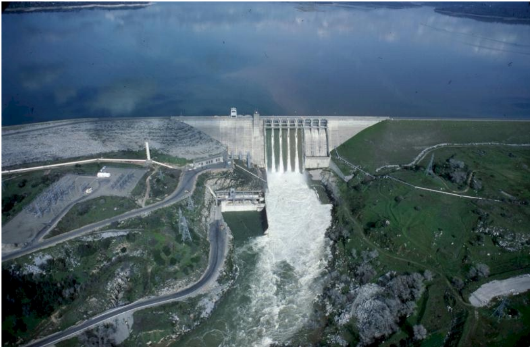
Photograph 5.1-I-13. Folsom Dam (Source: Bureau of Reclamation.)
