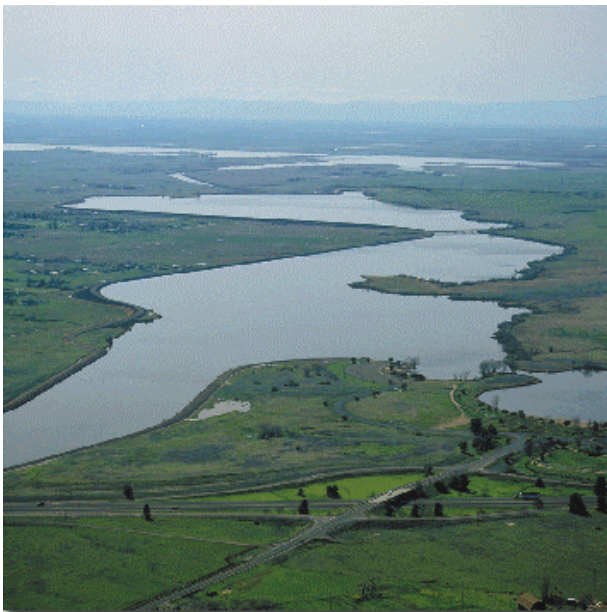
Photograph 5.1-9. Thermalito Forebay with Afterbay in Background (Source: California Department of Water Resources.)
