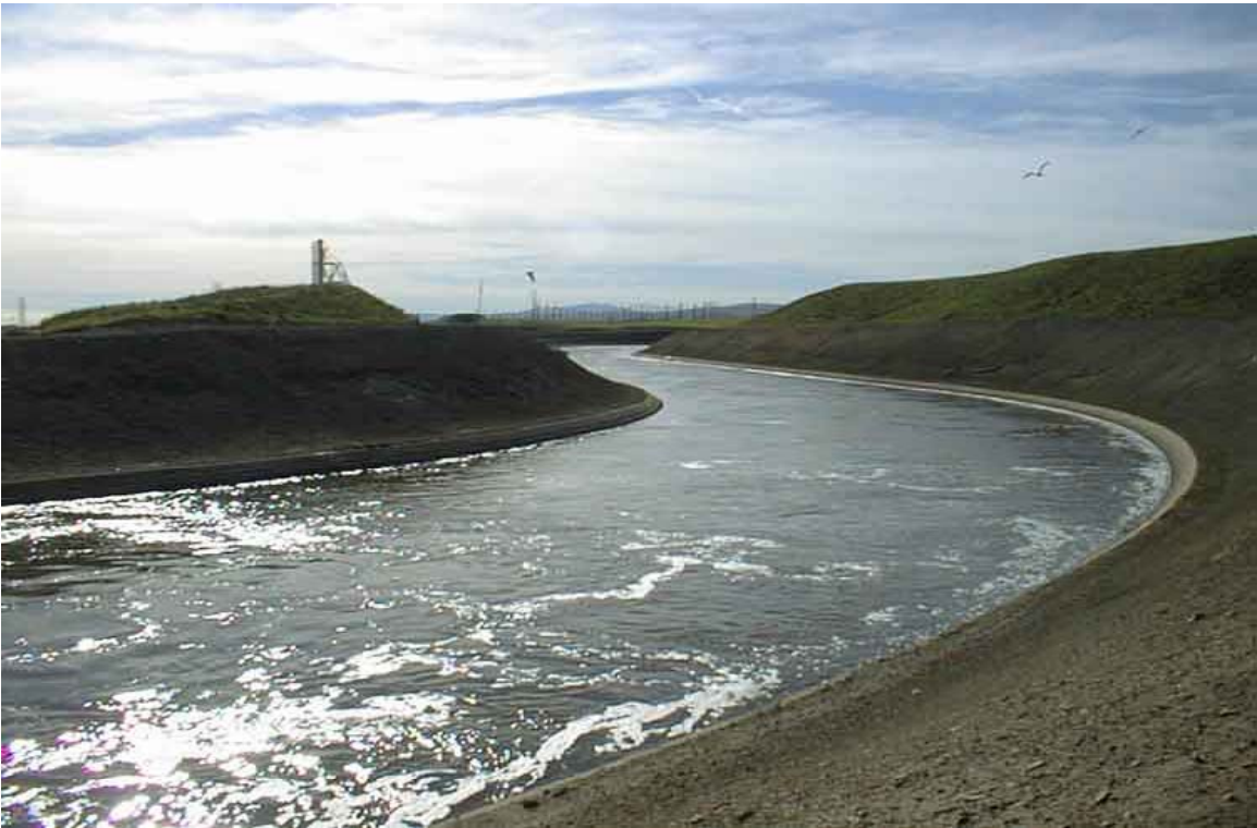
Photograph 5.1-16. CVP Delta-Mendota Canal at Mile 4.0 (Source: San Luis and Delta-Mendota Water Authority.)
