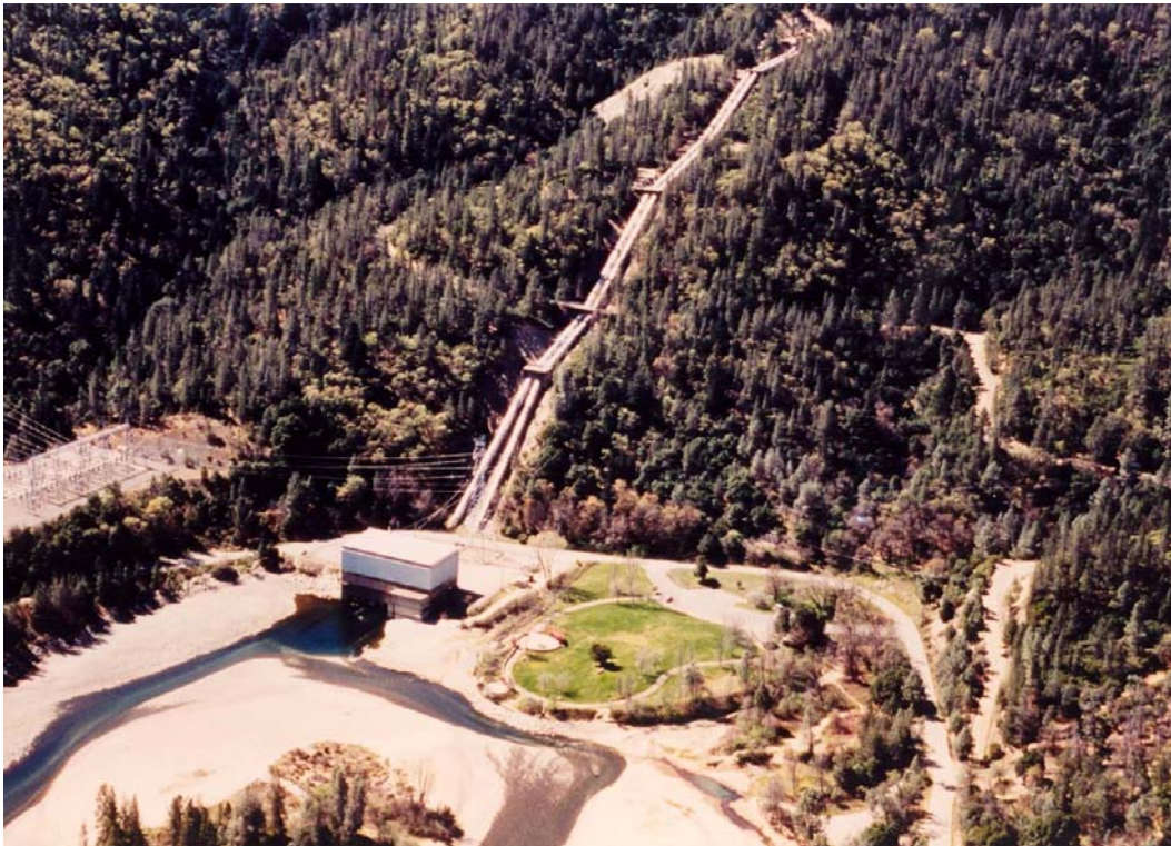
Photograph 5.1-3. Judge Francis Carr Powerplant (Source: Bureau of Reclamation.)
