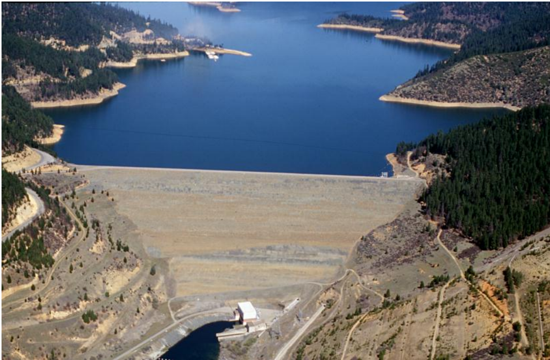
Photograph 5.1-1. Trinity Dam and Powerhouse (Source: Bureau of Reclamation.)
