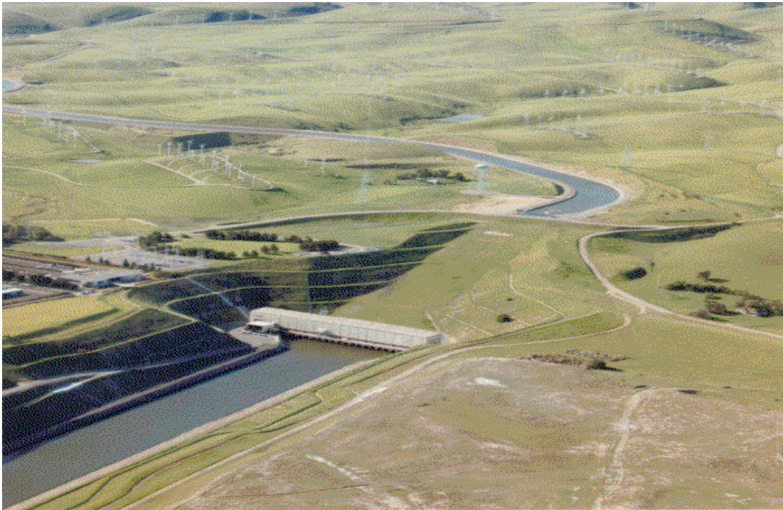
Photograph 5.1-17. SWP Harvey O. Banks Pumping Plant (Source: California Department of Water Resources.)
