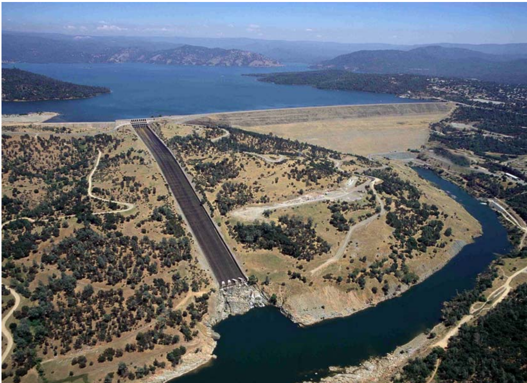
Photograph 5.1-7. Oroville Dam (Source: Bureau of Reclamation.)
