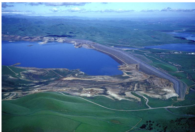
Figure 3.14-9. San Luis Reservoir and O'Neill Forebay
