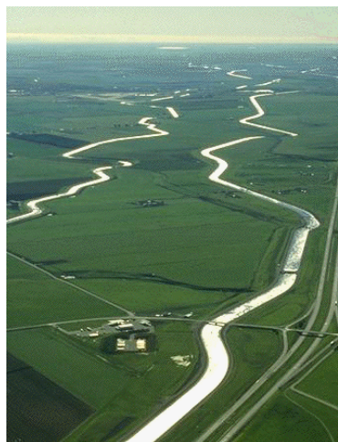
Delta-Mendota Canal and California Aqueduct
