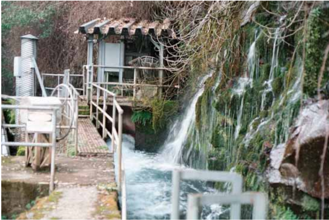
Figure 4.3-3. Spring Flow at Eagle Canyon Diversion Dam Flowing out of a Basalt Formation on the Southern Canyon Wall
