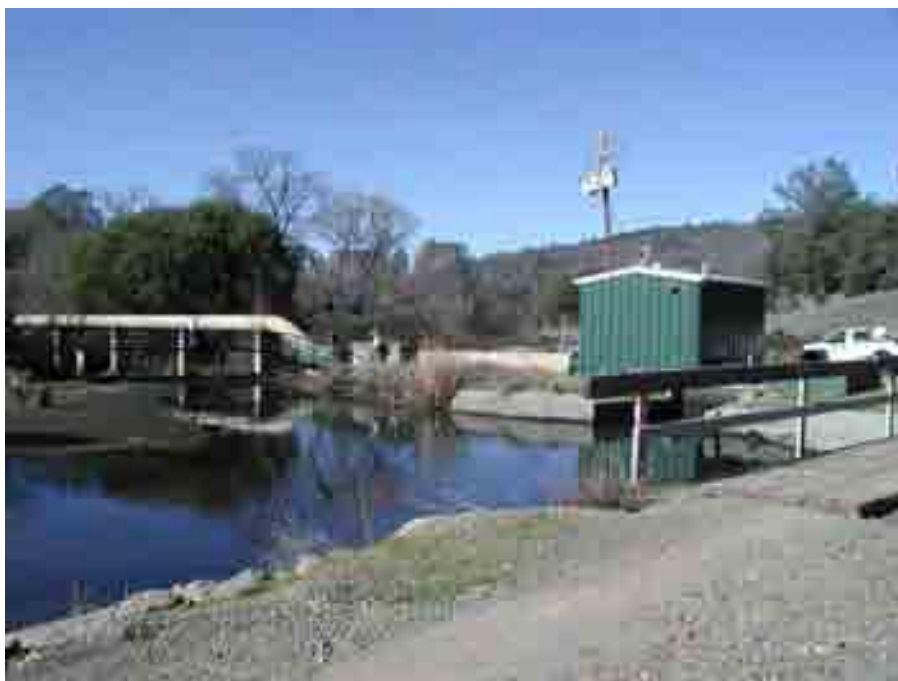
Figure 4.8-4 Asbury Pump Station
