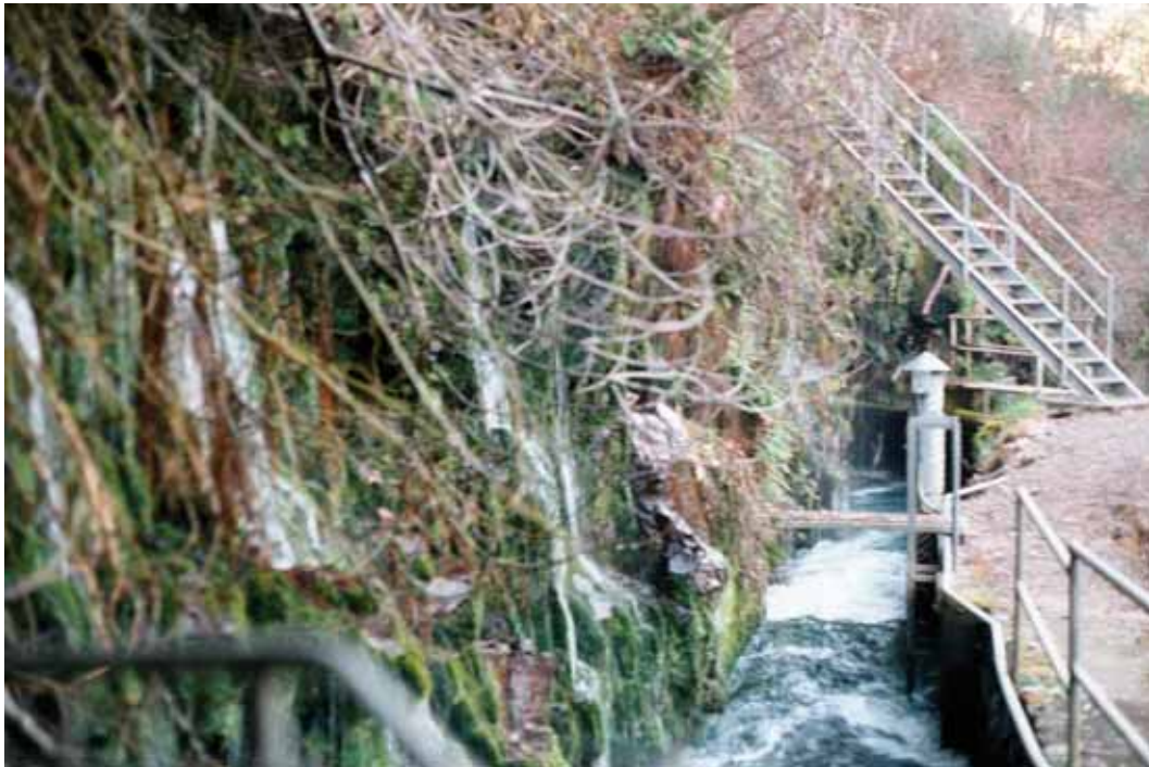
Figure 4.3-4. Spring Flow Entering Eagle Canyon Canal at Eagle Canyon Diversion Dam, Looking Downstream
