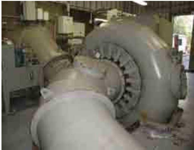
Volta 2 Powerhouse—Hydroelectric Turbine
