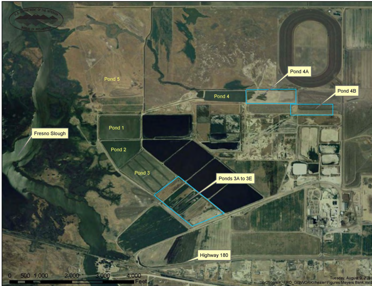
Figure 2-1 Existing Ponds at Meyers Bank
