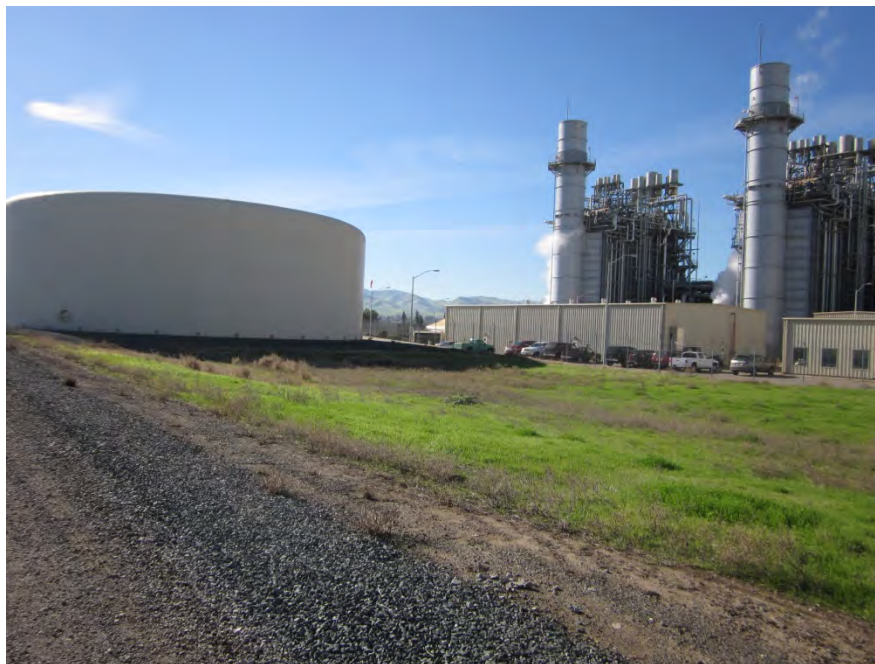
View looking south at an existing storage tank. The DEC is to the right (west)
