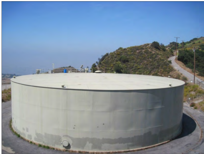
Figure 2-5: Example of a Recycled Water Storage Tank
