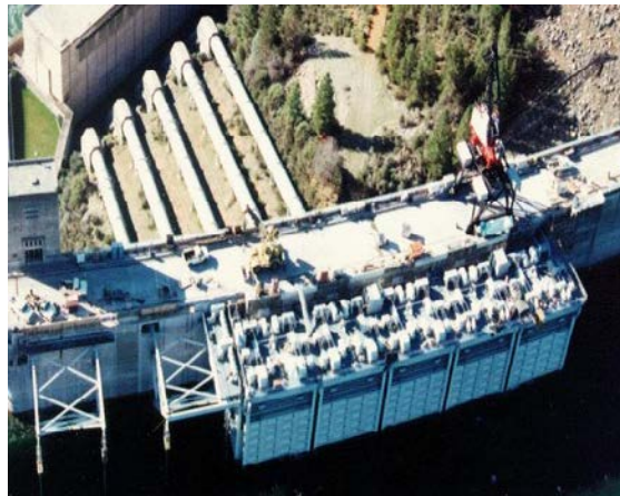
30 31 Figure 2-4. TCD Located on Upstream Face 32 of Shasta Dam
