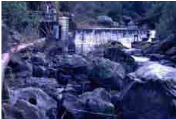
Wildcat Diversion Dam and Pipeline
