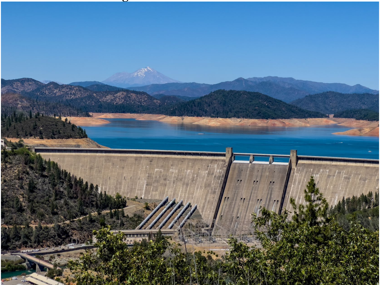
Shasta Dam and Lake on July 20, 2022. Photo Credit: Reclamation
