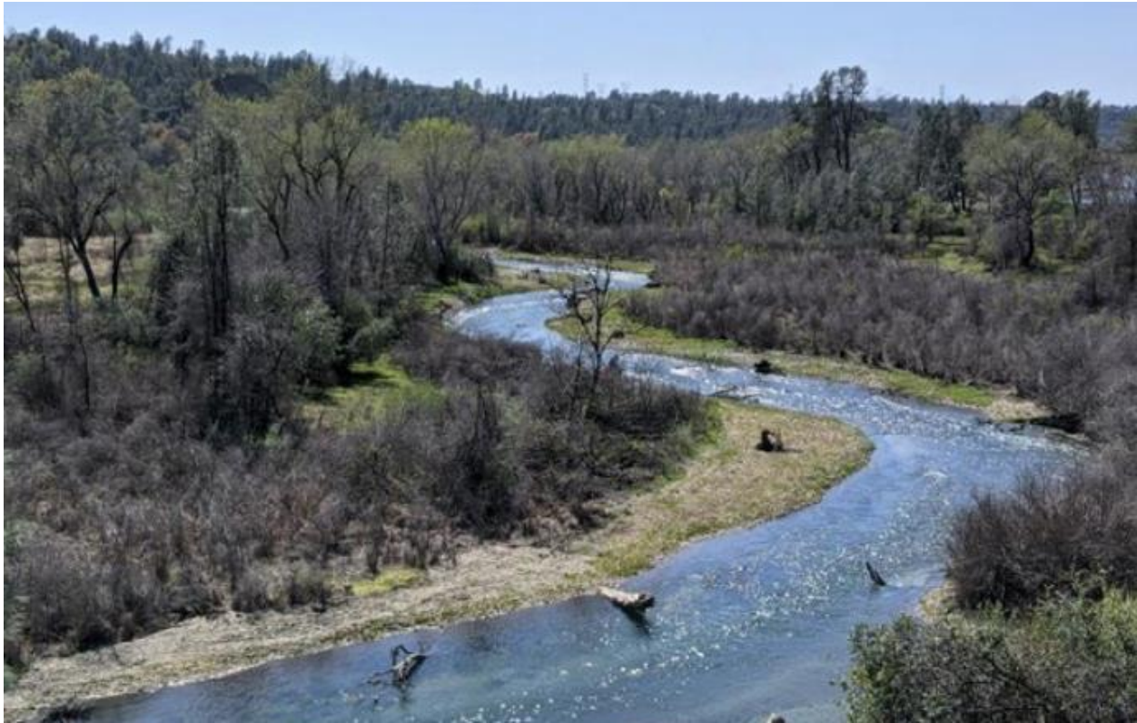
Figure 9. Clear Creek flowing through the Phase 3C stream channel restoration project area. Spring plant growth reveals that the revegetation efforts were successful on the newly created river bars. Photo credit: Derek Rupert, Bureau of Reclamation.
