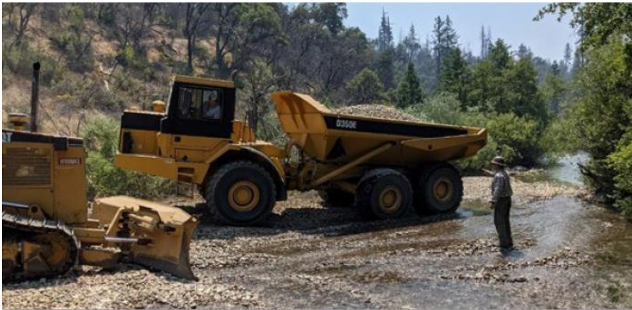
Figure 8. Implementation of the gravel augmentation project at the Below Dog Gulch site on Clear Creek. Photo credit: Derek Rupert, Bureau of Reclamation.
