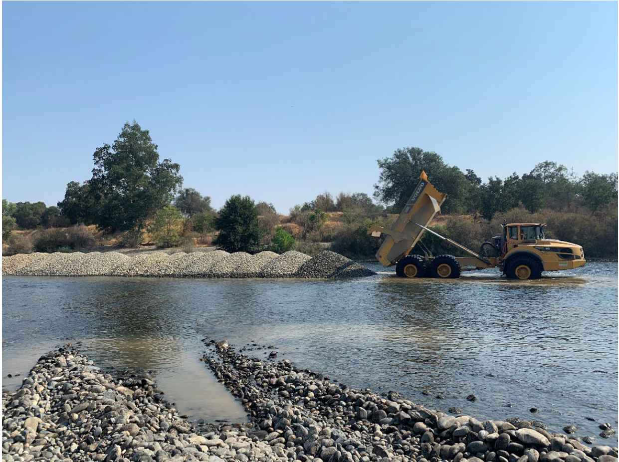
Figure 2. A dump truck placing sorted gravel into the mainstem American River.
