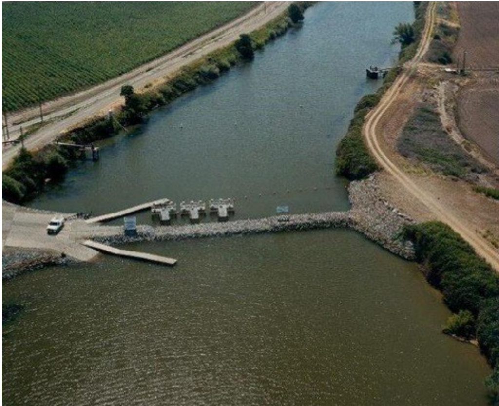
Figure 25. Agricultural barrier on Old River near Tracy, California. (DWR)
