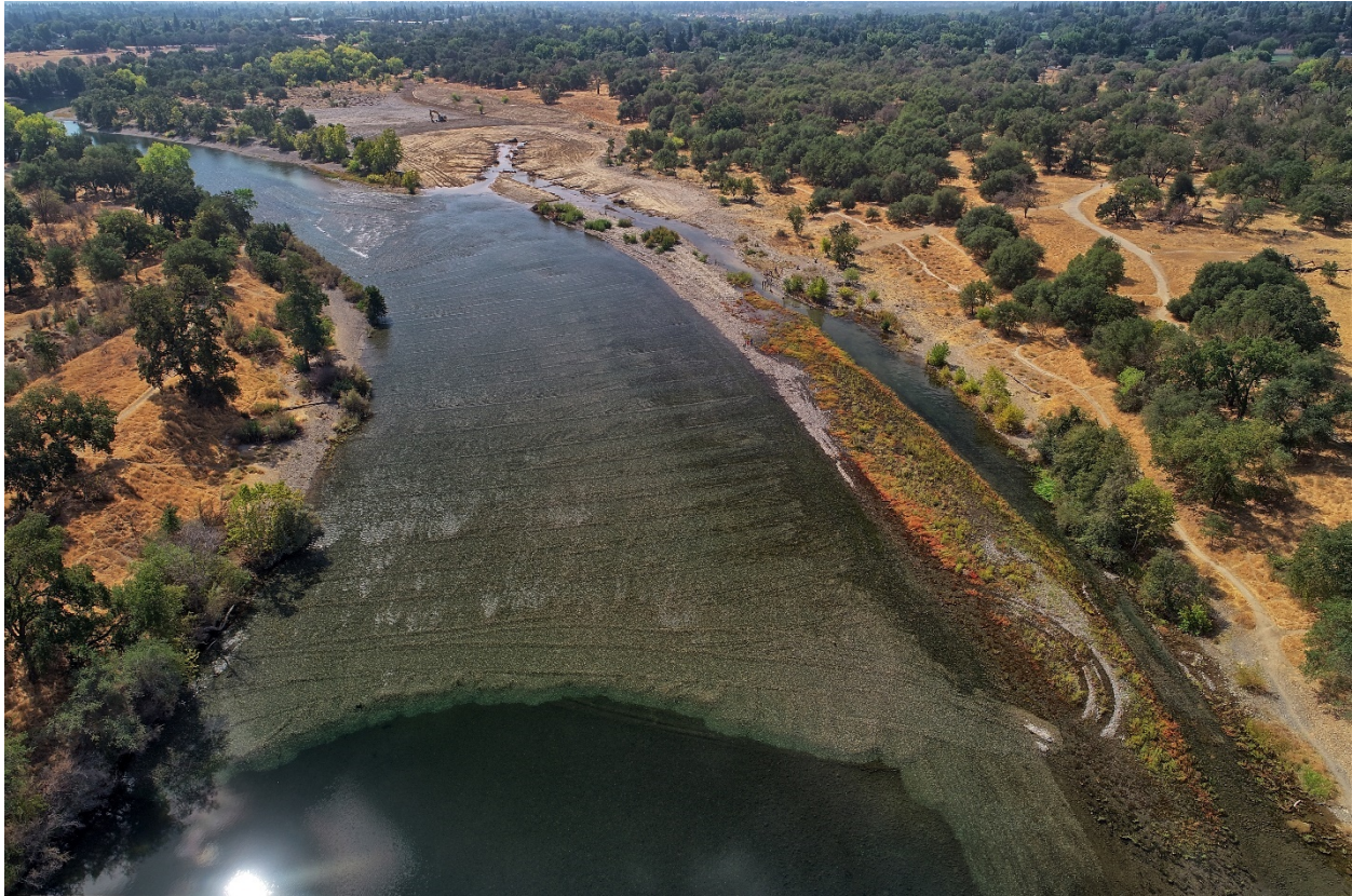
Figure 10. Looking downstream at completed construction at Ancil Hoffman.
