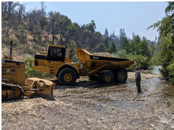
Figure 7. The 2021 gravel augmentations at Dog Gulch. This riffle supplementation-style augmentation produces immediate spawning habitat and improve floodplain inundation. Six large boulders were incorporated into the site.
