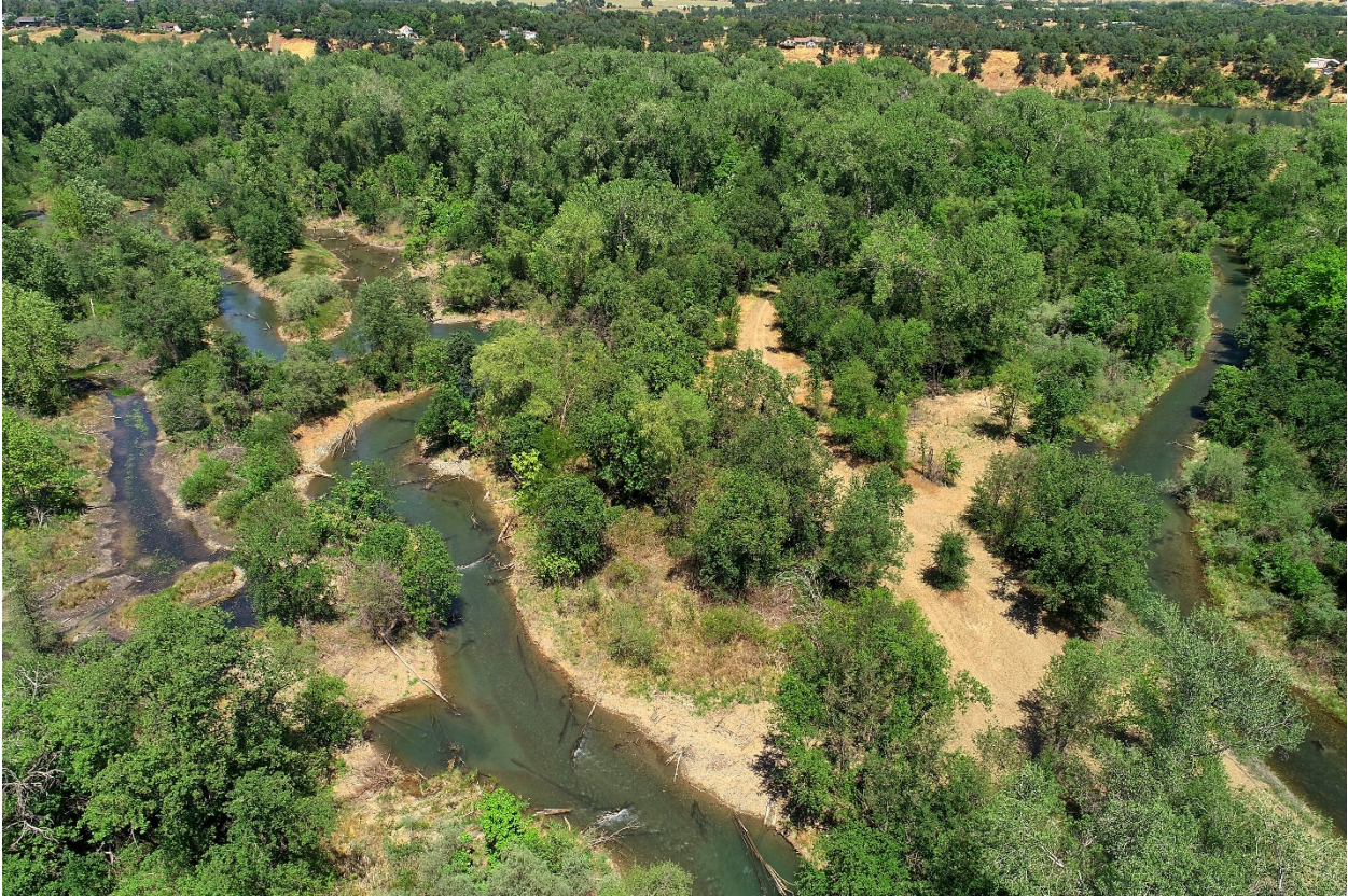
Figure 3. Looking upstream at the Anderson River Park Side Channels project with phase I channel on the right and phase II channel on the left.
