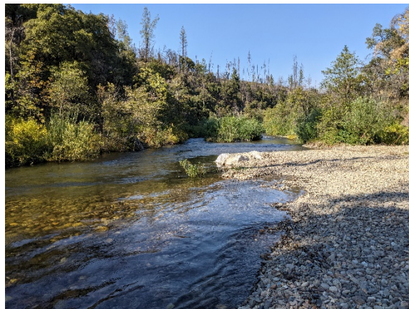
Figure 7. The 2021 gravel augmentations at Dog Gulch. This riffle supplementation-style augmentation produces immediate spawning habitat and improve floodplain inundation. Six large boulders were incorporated into the site.
