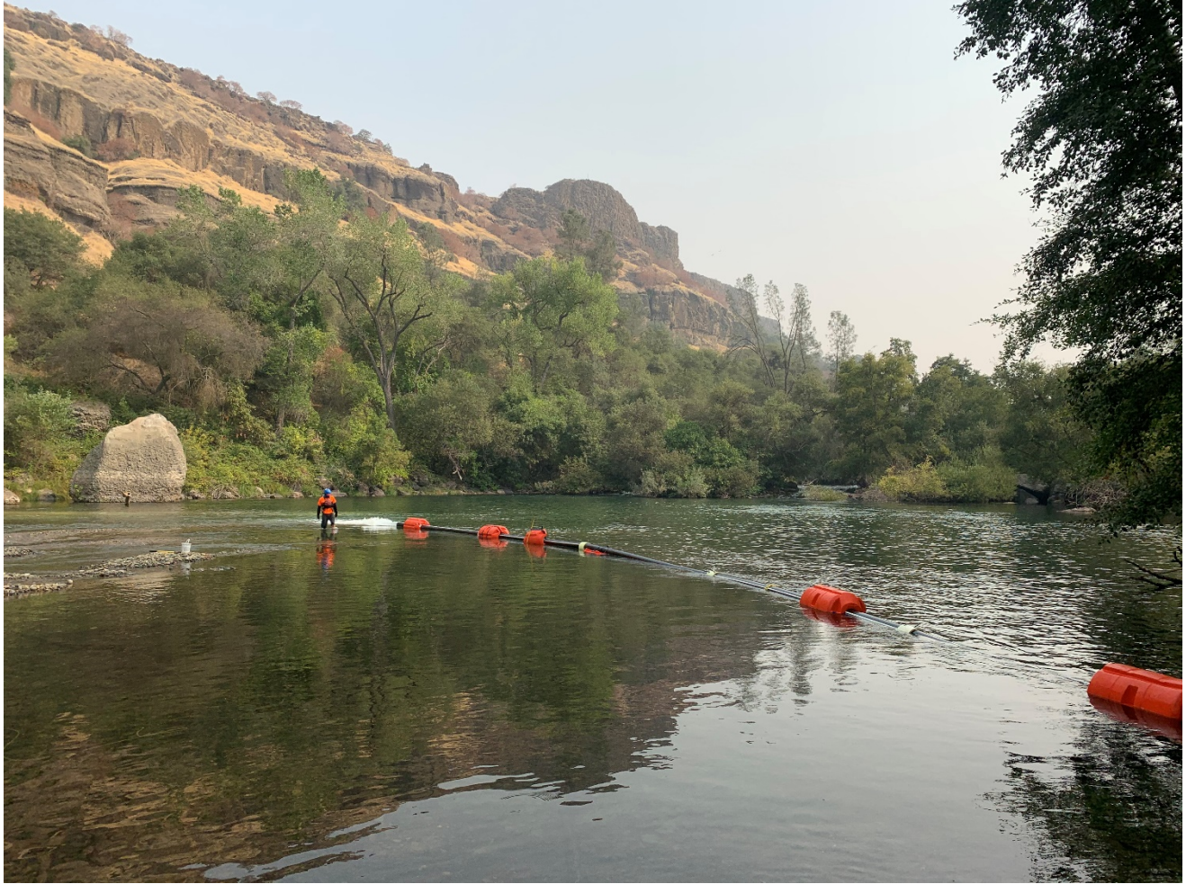
Figure 5. Salmonid spawning gravel injection project at the Goodwin Dam Recreation Area on the Stanislaus River. (Photo credit: Elissa Buttermore, Reclamation)
