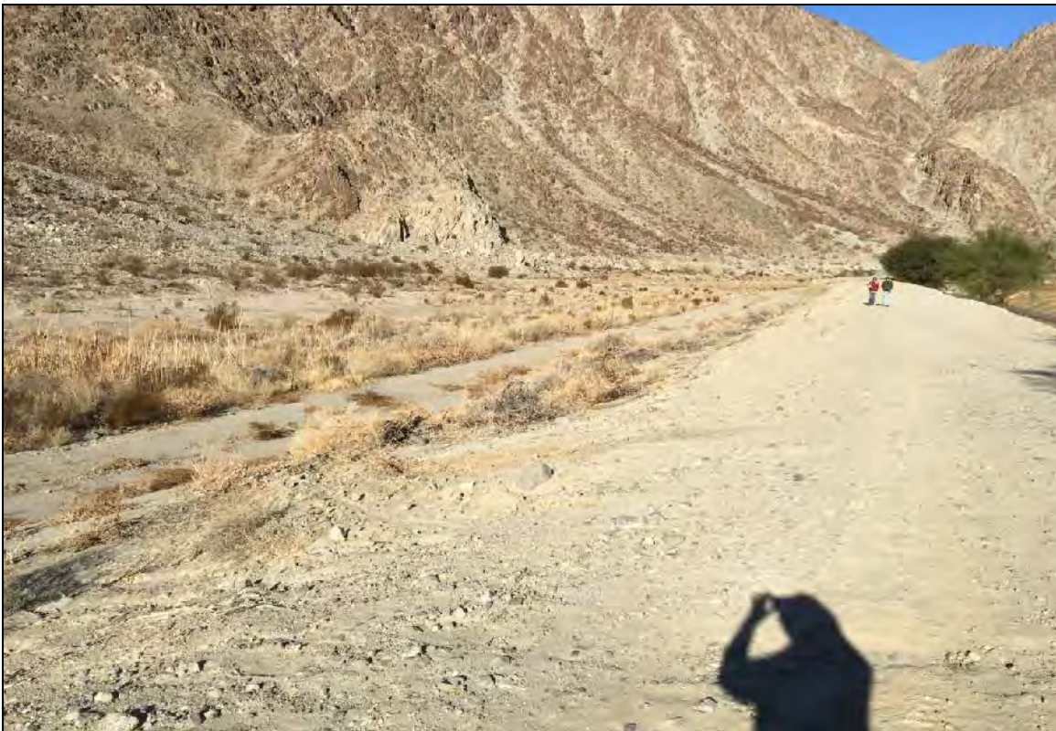
Photo 4. Proposed alignment of PBS barrier along the east-central portion of alignment (adjacent to PGA West Golf Club). View facing northwest.
