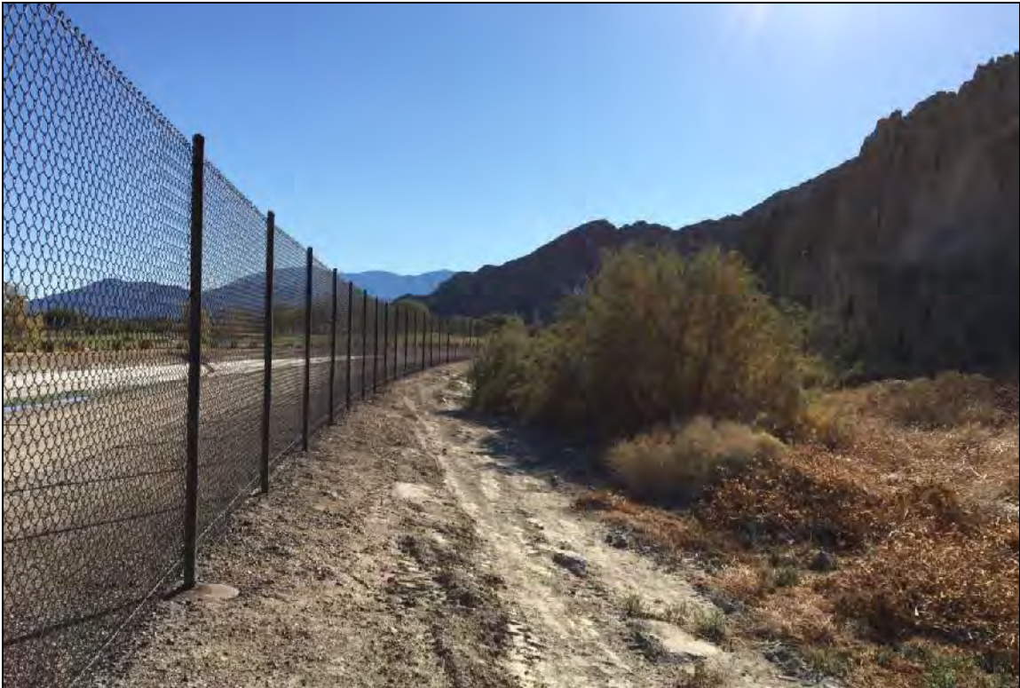
Photo 10. Proposed alignment of PBS barrier along the east-central portion of alignment (adjacent to the existing Coachella Branch of the All American Canal fence). View facing SE.
