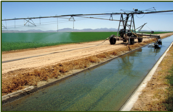
Low-pressure sprinkler irrigation Source: Bureau of Reclamation
