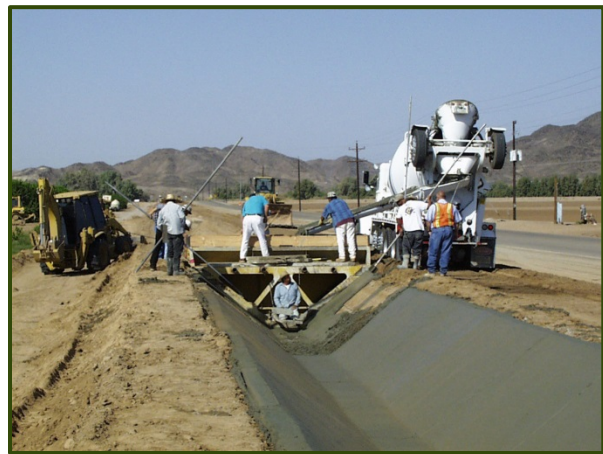
Dome Canal lining
