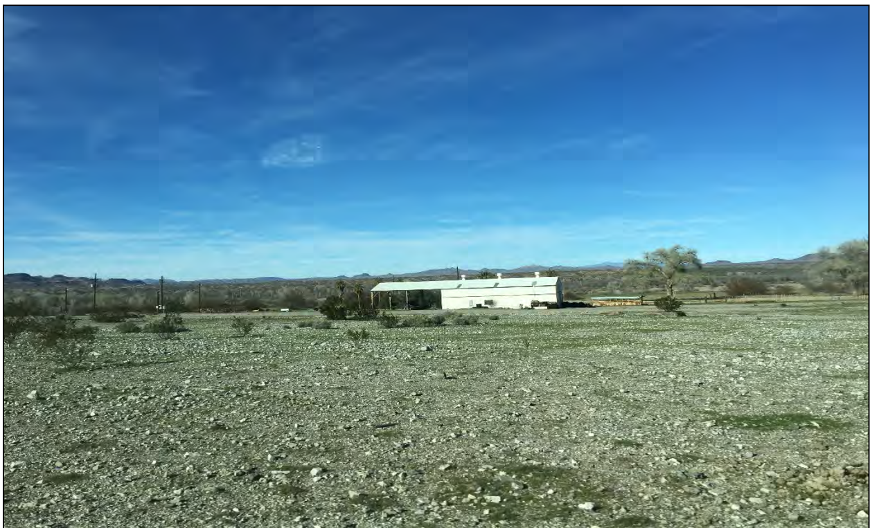
Figure 23. Planet Ranch Buildings (2017).
