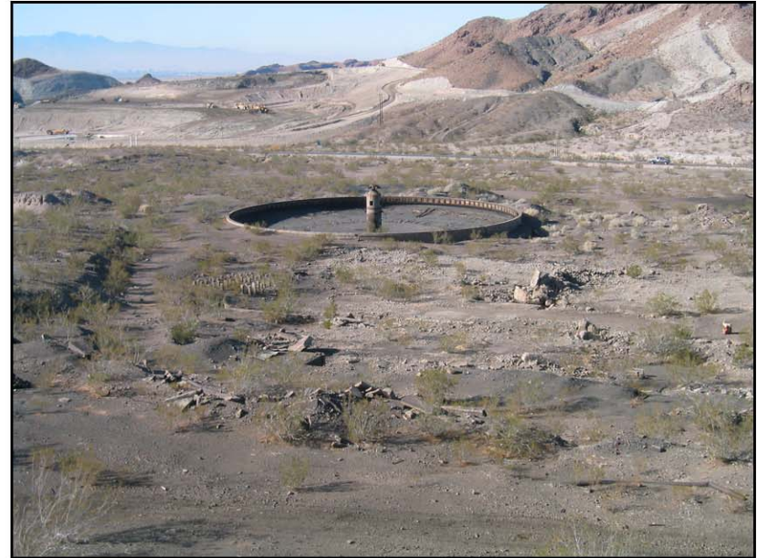
Photo 14 – Mill building foundations, conditioner piers, and thickener facing NW. December 1, 2006.
