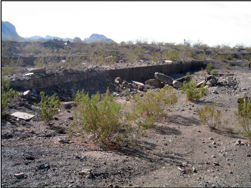
Photo 13 – Mill site foundations facing SW, July 11, 2006.
