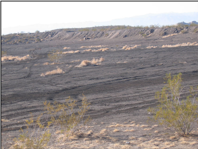
Photo 27 – Tailings pond 3 facing NW. Dust palliative deteriorated due to high OHV traffic. January 9, 2007.
