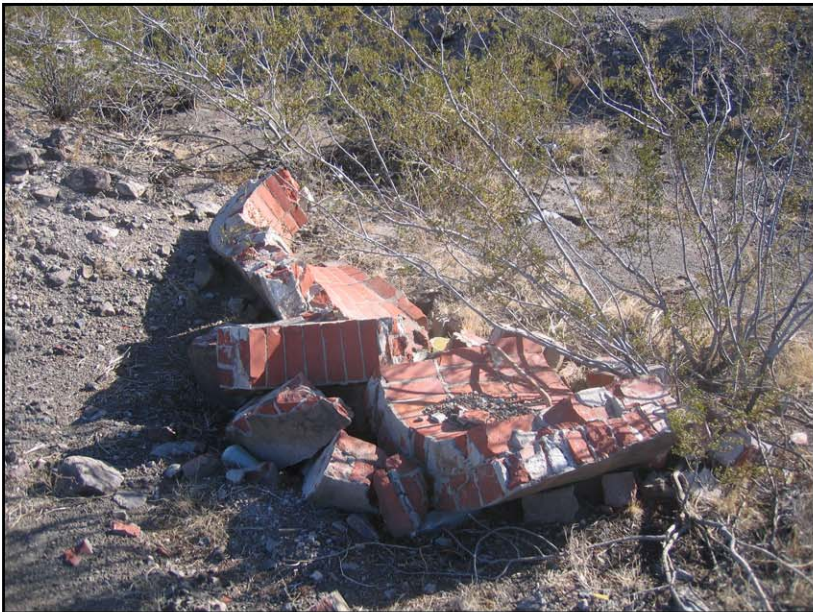
Photo 23 – Remains of brick sewer line interceptor, mill site area. January 9, 2007.
