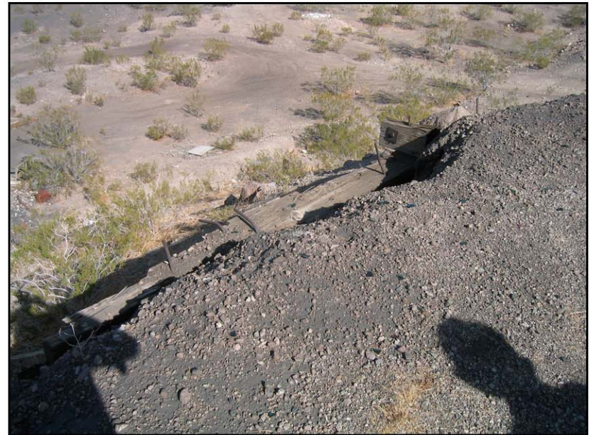
Photo 8 – Former ore hopper location facing down and NE. July 11, 2006.
