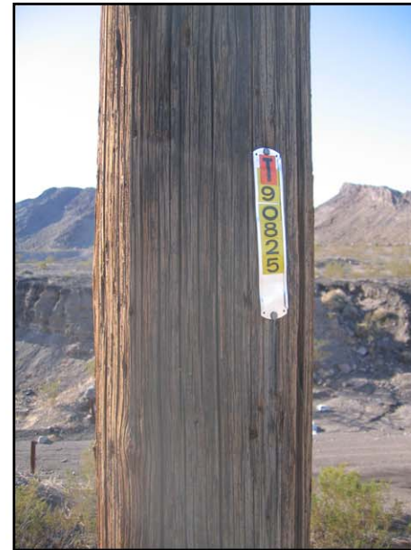
Photo 32 – Pole number on BMI control line, N of B Pit mine haul road. January 9, 2007.
