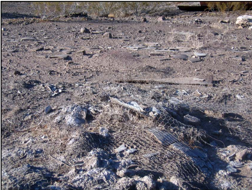
Photo 35 – Weathered transite asbestos and apparent friable asbestos between thickeners and N edge of Hydro Pit. January 9, 2007.
