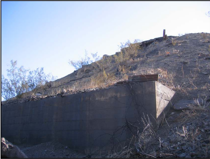
Photo 9 – Former ore hopper location facing up and SE. January 9, 2007.
