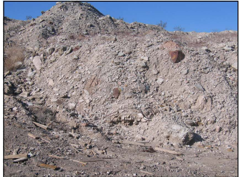
Photo 40 – Buried drums and solid waste NW of Hulin Pit facing N. January 23, 2007.
