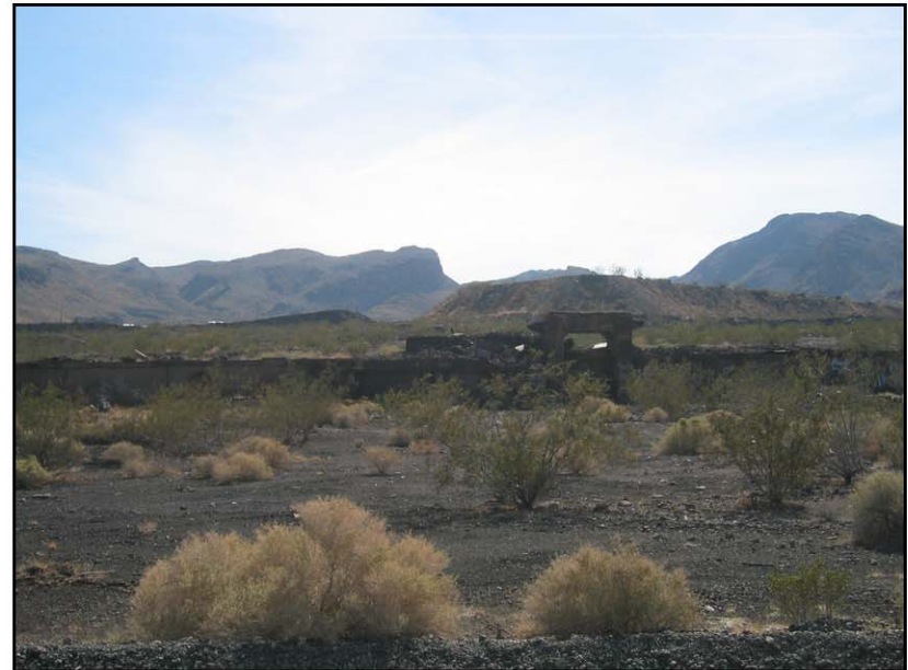
Photo 16 – Nodule stockpile area with kiln foundation behind facing S. July 11, 2006.
