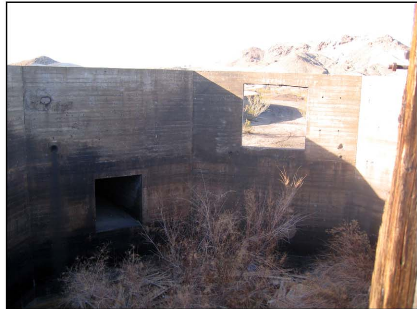
Photo 20 – East octagonal sump interior, approximately 15 ft fall, facing N. January 9, 2007.
