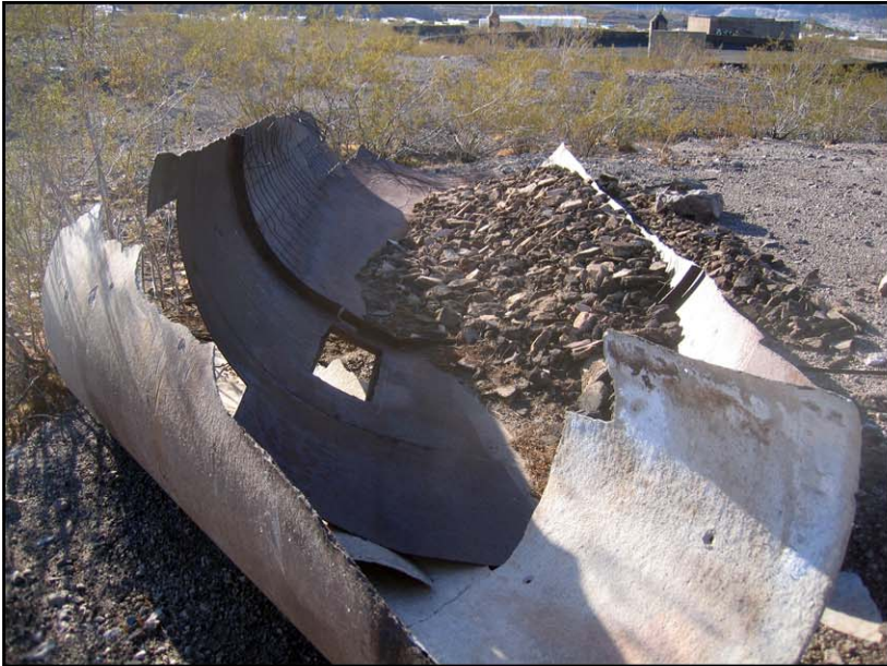
Photo 33 – Weathered transite asbestos containing material, between thickeners and N edge of Hydro Pit facing W. January 9, 2007.
