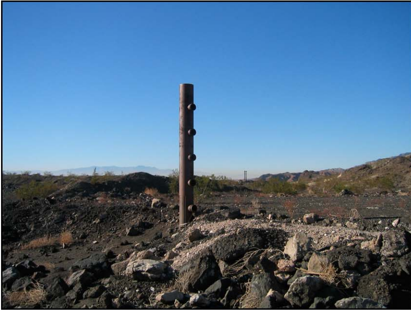
Photo 29 – Tailings waste pipe, tailings pond 1, facing NW. July 11, 2006.
