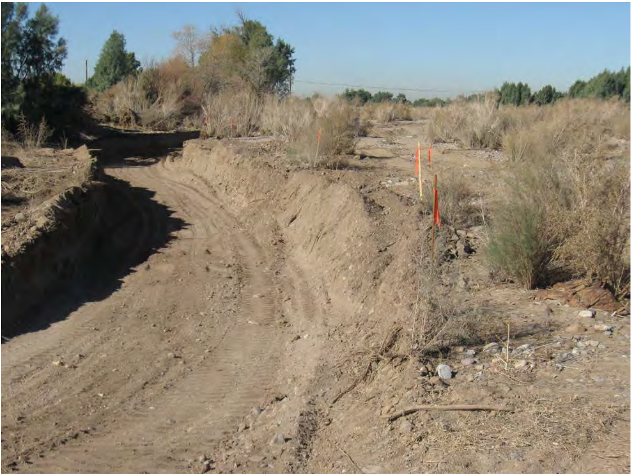
Photo 3. – Completion of Channel 1 Excavation.
