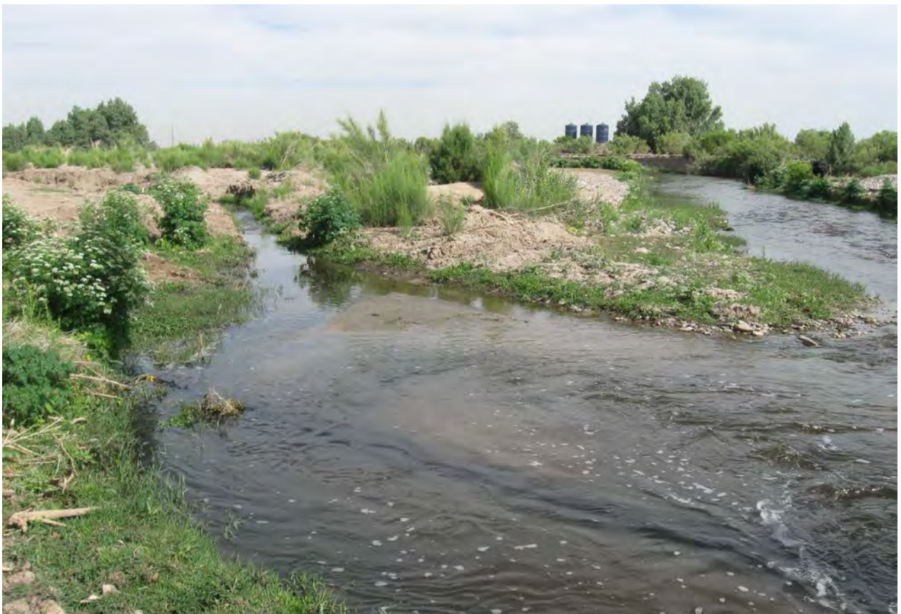
Photo 7. – Looking Downstream at the Diversion from the SCR Flow Channel (on Right) into the ERDP (on Left).
