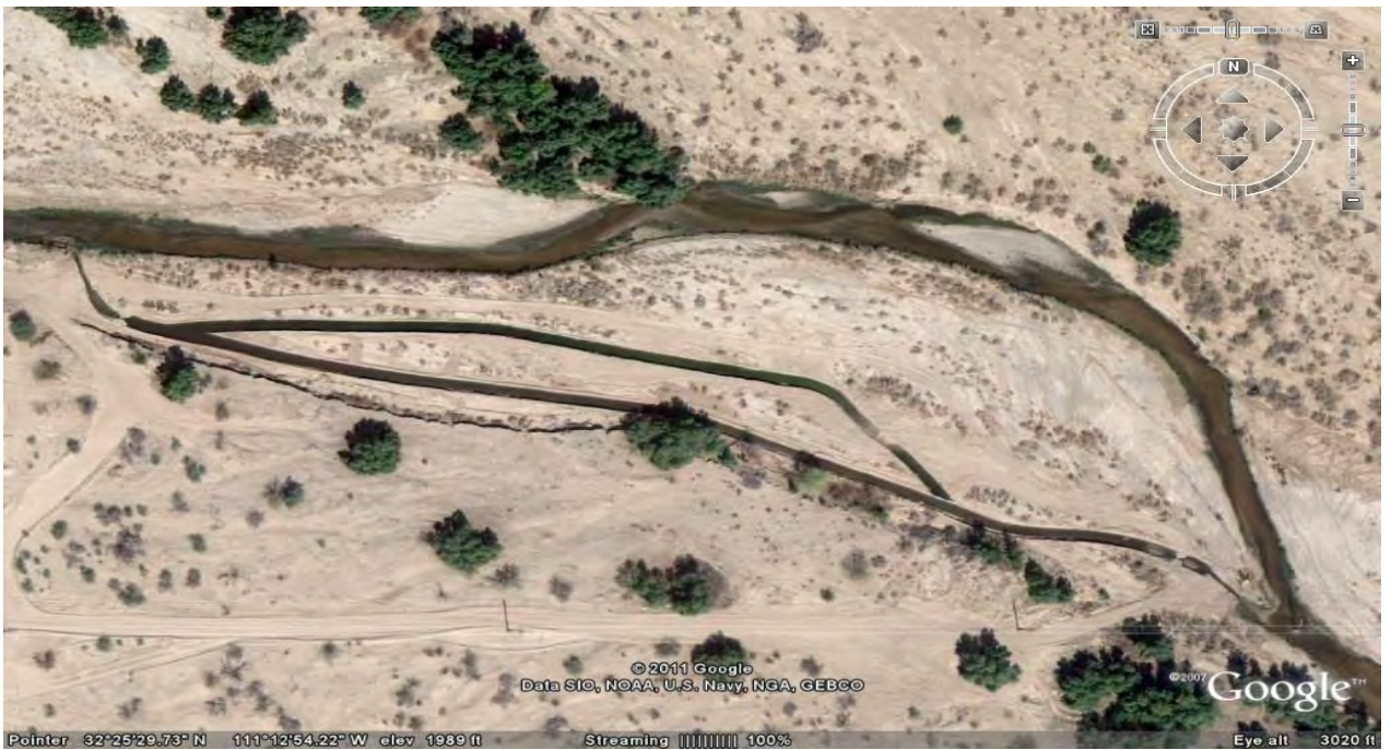
Photo 11. – Aerial Image of Constructed ERDP.
