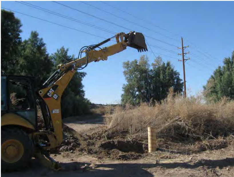
Photo 4. – Placement of Concrete Anchor for Upstream Flume.
