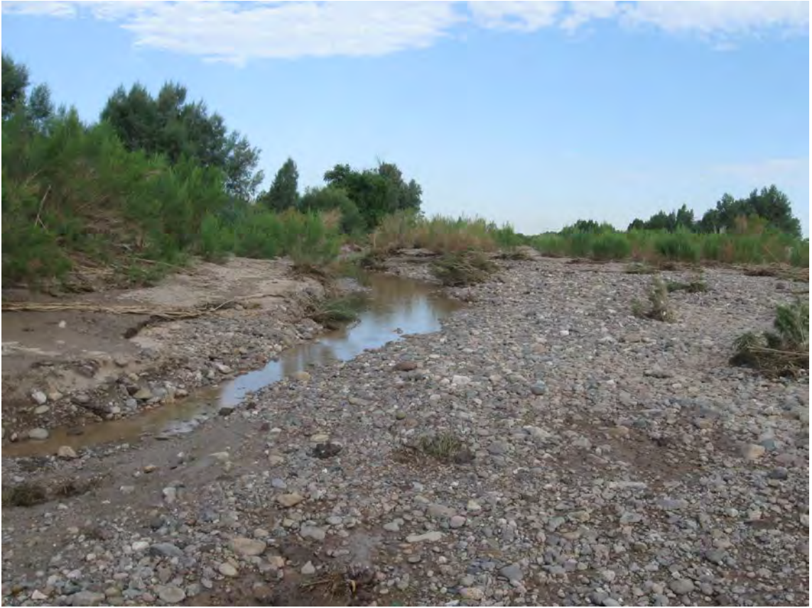
Photo 16. – Looking Downstream at Channel 1 and Buried Upstream Flume after July 5 th and 6 th Stormflows Washed Out Project.
