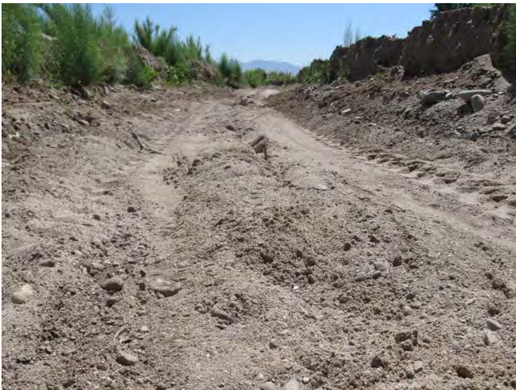
Photo 13 – Channel 2 after Drying, Scraping, and Ripping during Maintenance Event 1.
