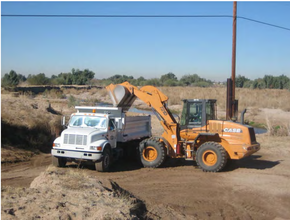
Photo 2. – Removal of Excavated Material during Excavation.
