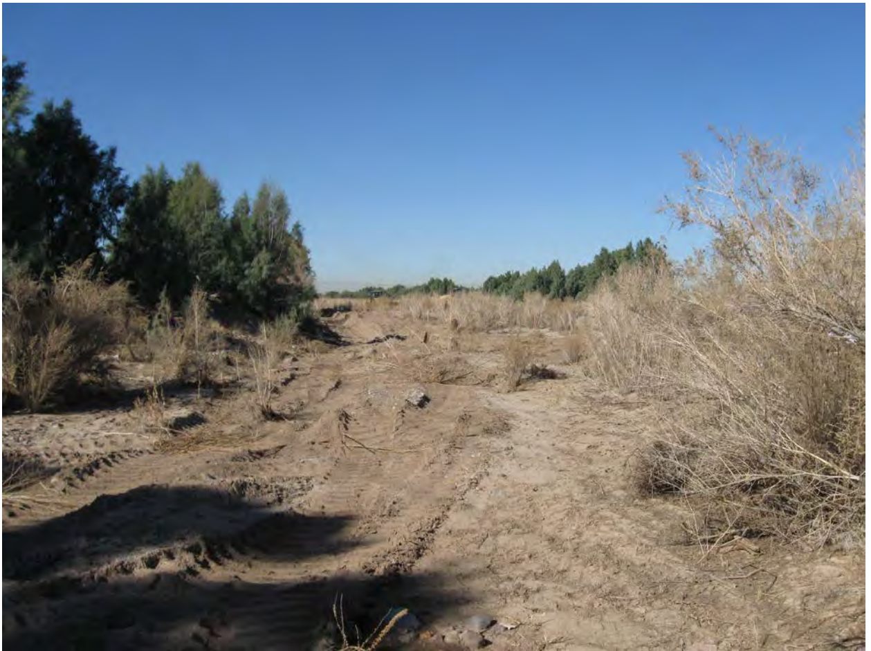
Photo 1. – Vegetation Cleared and Start of Excavation in Channel 1.
