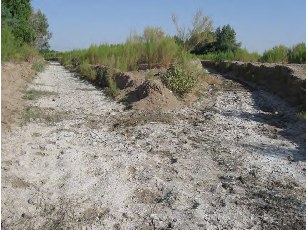
Photo 15. – Looking Downstream at the Divergence between Channels 1 and 2 after Drying during Third Maintenance Event.
